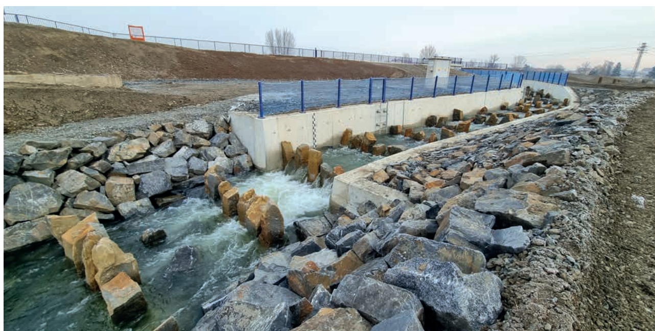
Reconstruction of the Hranice Weir – Fish ladder (Source: Morava River Board, s.e.)
