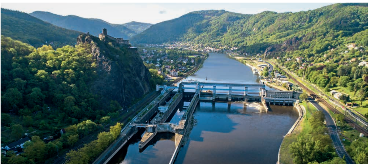
The Lock Chamber Střekov (Source: Elbe River Board, s.e.)
