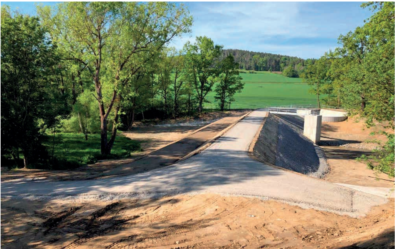
The Bavorovský Stream, small water reservoir Bavorov – reconstruction and de-mudding – condition after repair (Author: Bušek Jan)
