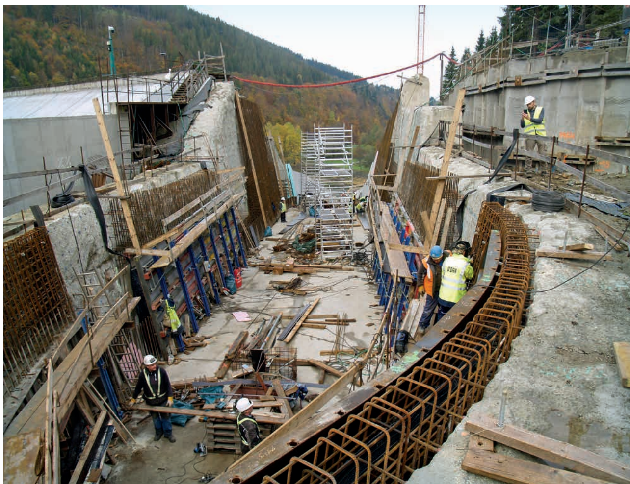
The Morávka Reservoir (Source: Oder River Board, s.e.)
