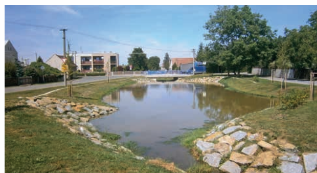
Flood control measure on the Markovický Stream (Source: Morava River Basin, s.e.)
