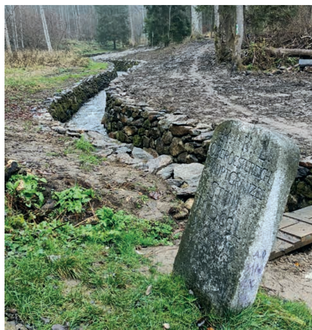
Fortification of the watercourse bed Světlá Stream, Český Krumlov District (Source: Forests of the Czech Republic, s.e.)
