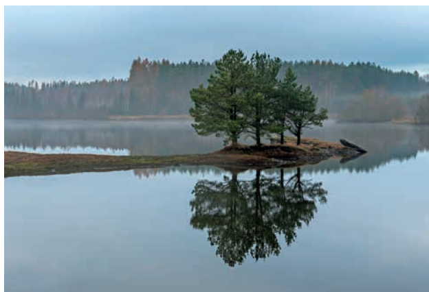
Drinking water reservoir Hamry (Source: Elbe River Board, s.e.)
