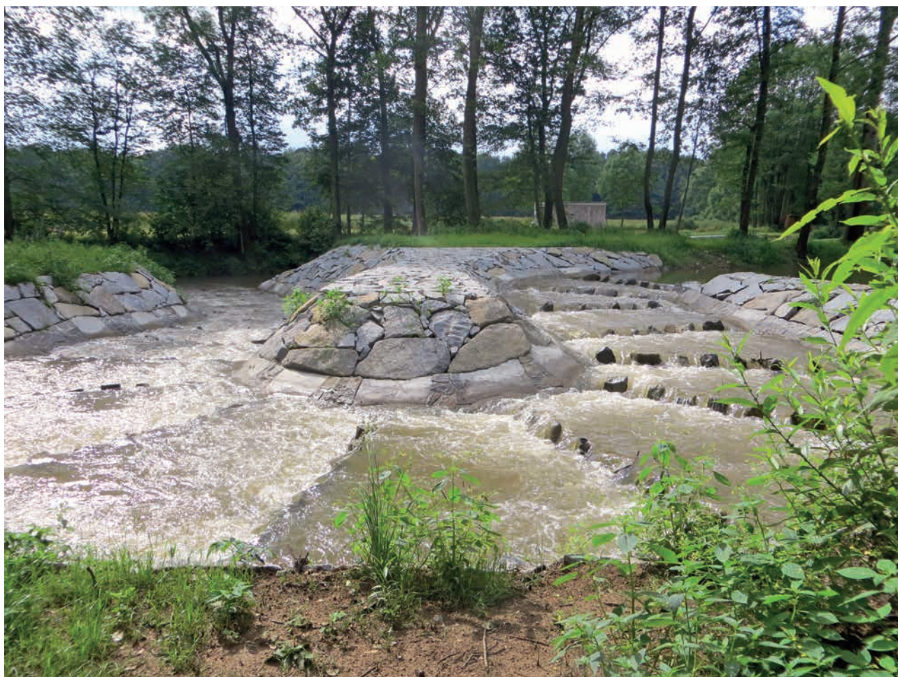
The Bystřice Weir on the Úhlava Stream (Source: Vltava River Board, s.e.)
