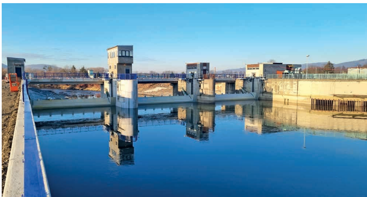
Reconstruction of the Hranice Weir (Source: Morava River Board, s.e.)
