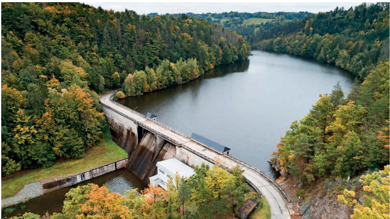
Drinking water reservoir Křižanovice (Source: Elbe River Board, s.e.)
