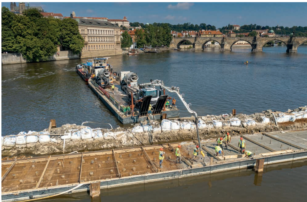
Old Town Weir, concreting (Source: Vltava River Board, s.e.)
