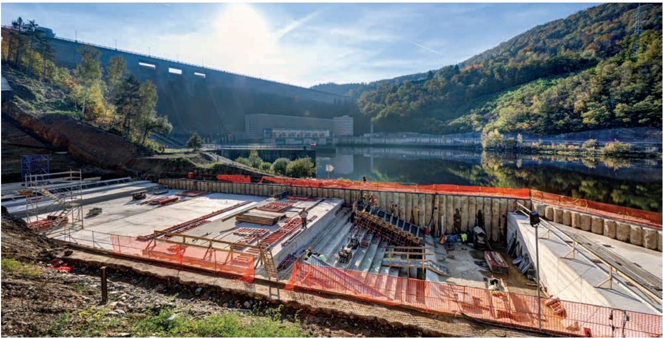
The Orlik Reservoir, realization of the test block of concreting (Source: Vltava River Board, s.e.)
