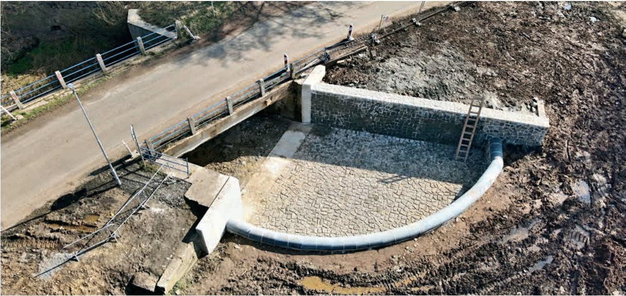
Finkl's Pond (source: Ohře River Board, s.e.)
