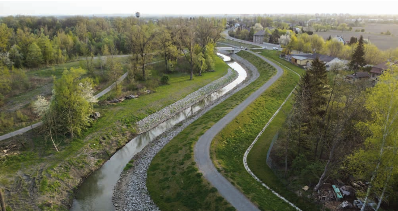
Completed section of the Pudlovská dike in Bohumín (source: Oder River Board, s.e.)
