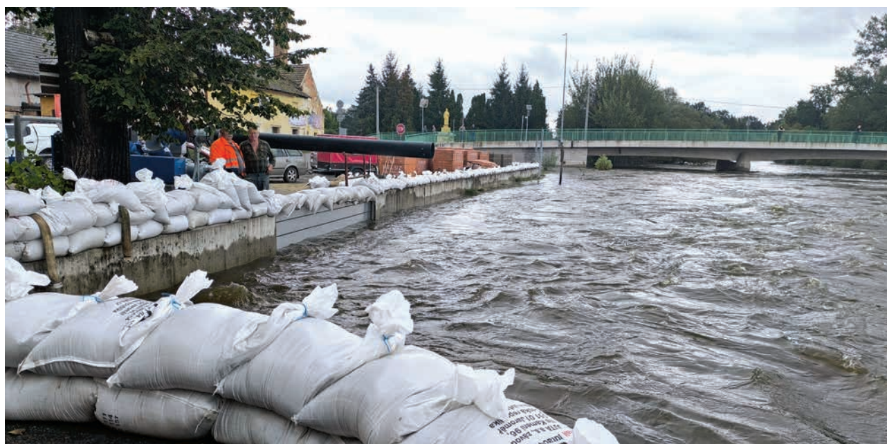
The Flood Control Measures (source: Vltava River Board, s.e.)
