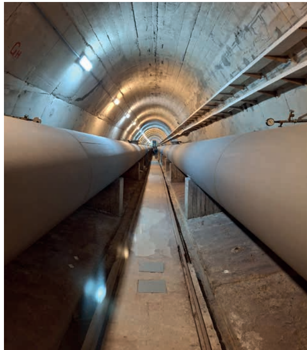
Tunnel at the Morávka Reservoir (author: Hubalová Petra)
