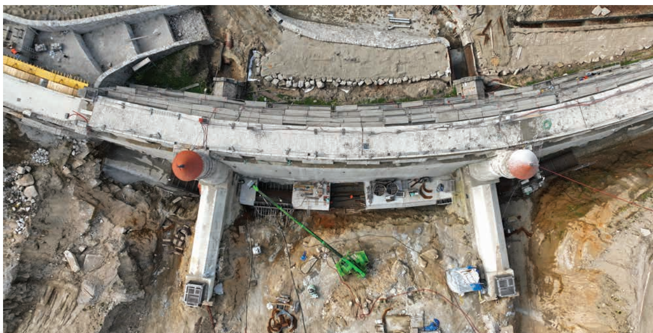
The Harcov Reservoir, injection (source: Elbe River Board, s.e.)
