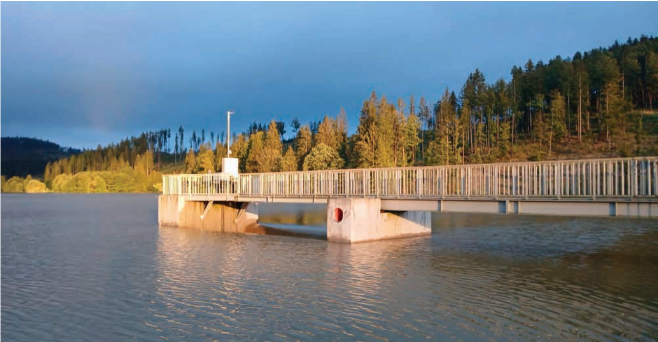
Flood dry reservoir Jelení on Kobyli Creek in Karlovice in operation (source: Odra River Board, s.e.)
