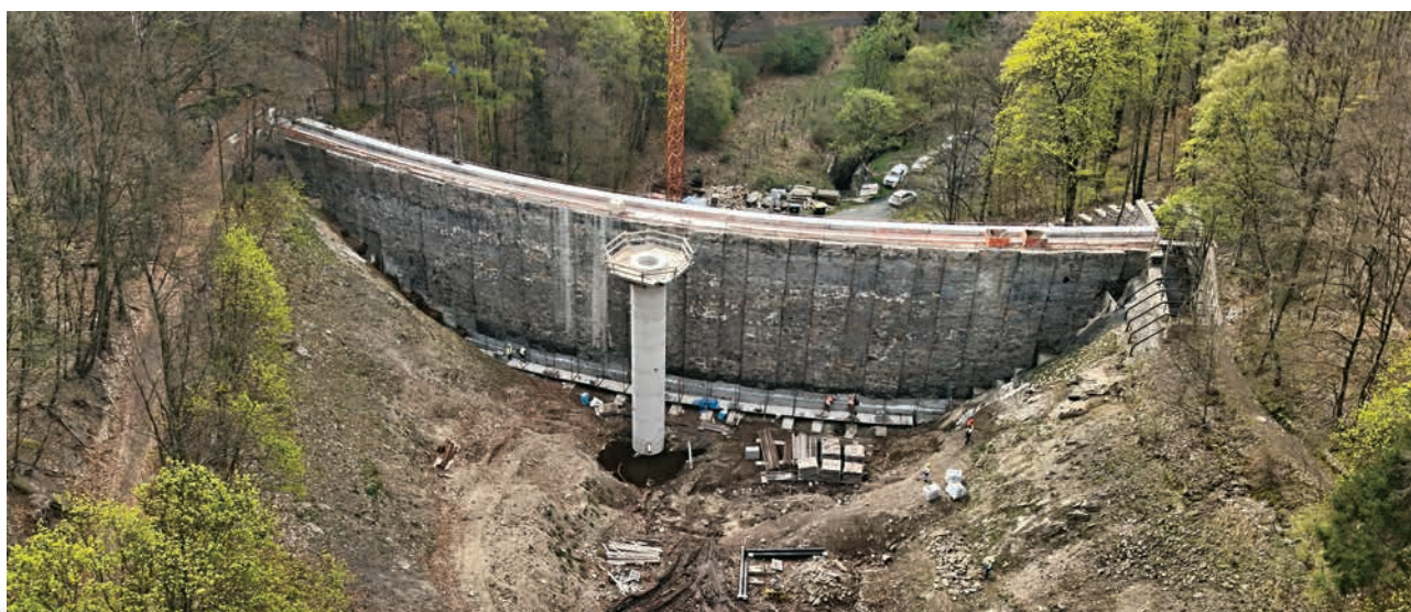
The Jezeří Reservoir, renovation (source: Ohře River Board, s.e.)
