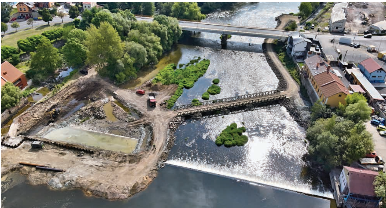
The Kadaň Weir, Renovation (source: Ohře River Board, s.e.)
