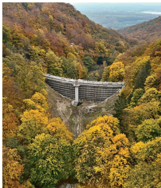
The Jezeří Reservoir (source: Ohře River Board, s.e.)
