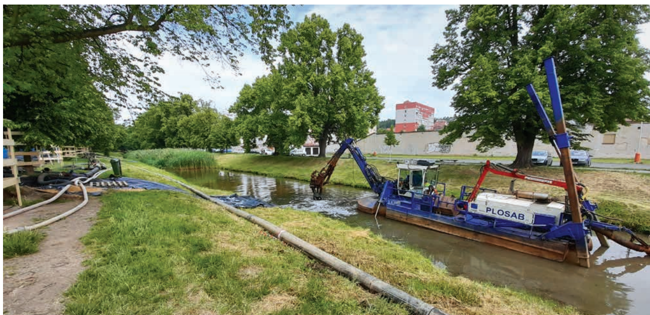
Rakovnický Stream, Rakovník, removal of sediment from the riverbed (source: Vltava River Board, s.e.)
