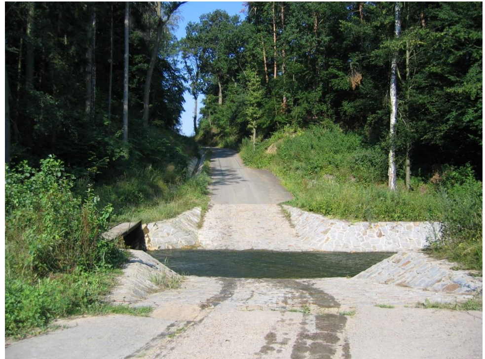
After realization – cadastre unit Skryje (district Havlíčkův Brod)
