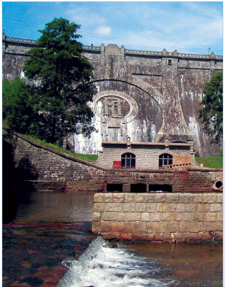
Labská water reservoir - Elbe river basin
