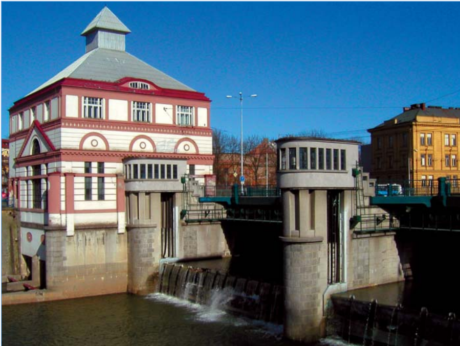
Moravia weir at Hradec Králové - Elbe river basin
