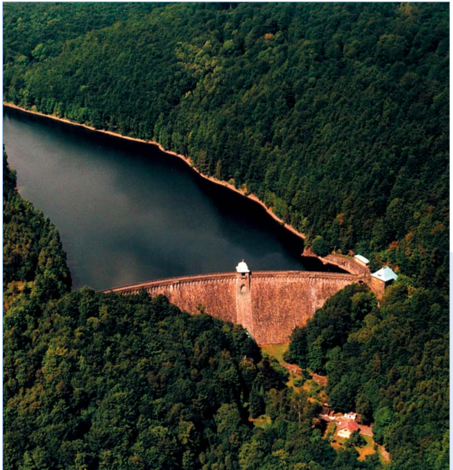
Janov water reservoir - Ohře river basin
