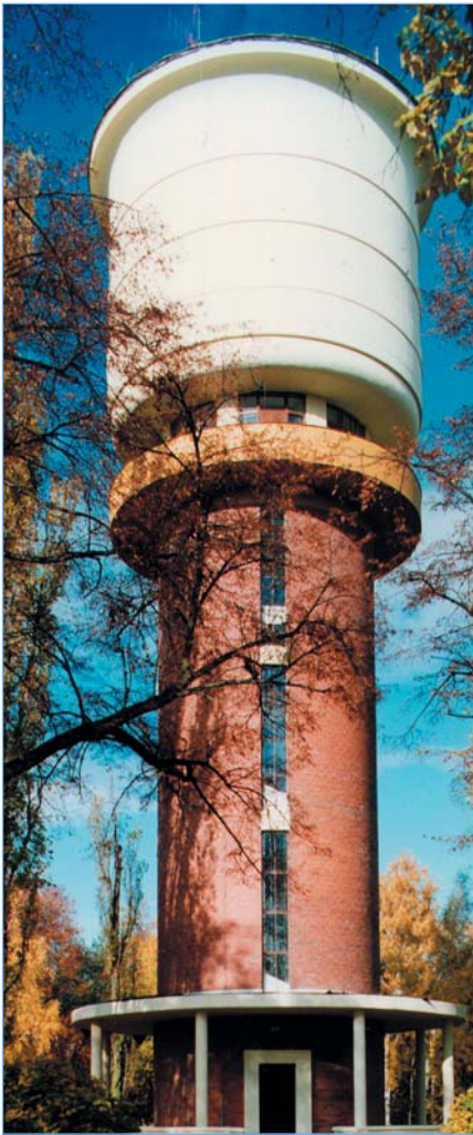
Distribution reservoir at Hradec Králové
