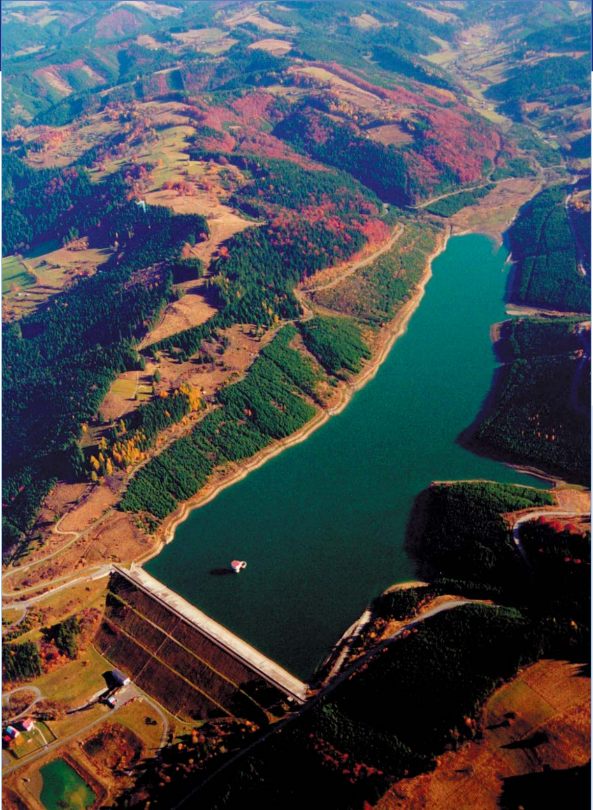
Karolinka water reservoir - Morava river basin
