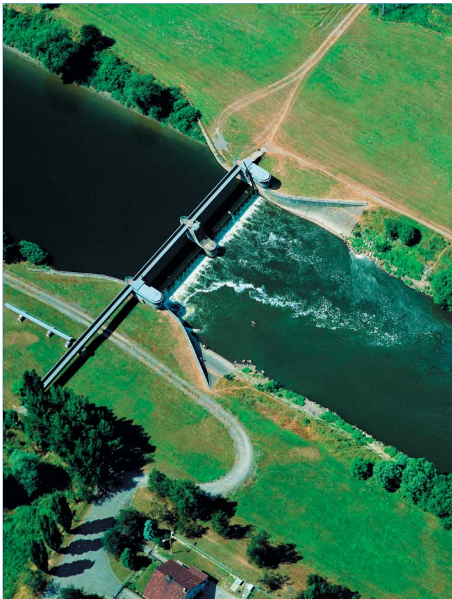
Lhotka weir - Odra river basin
