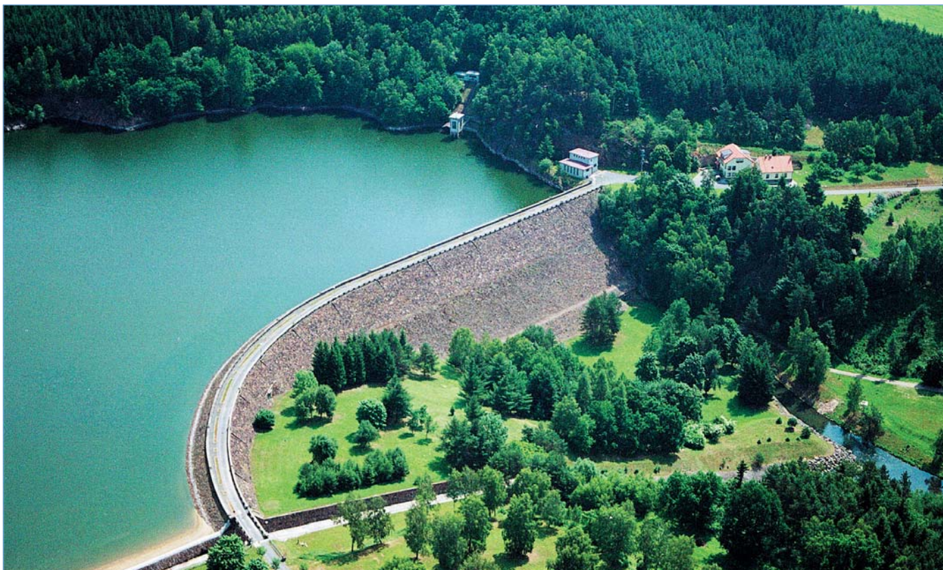
Mostišťe water reservoir - Morava river basin
