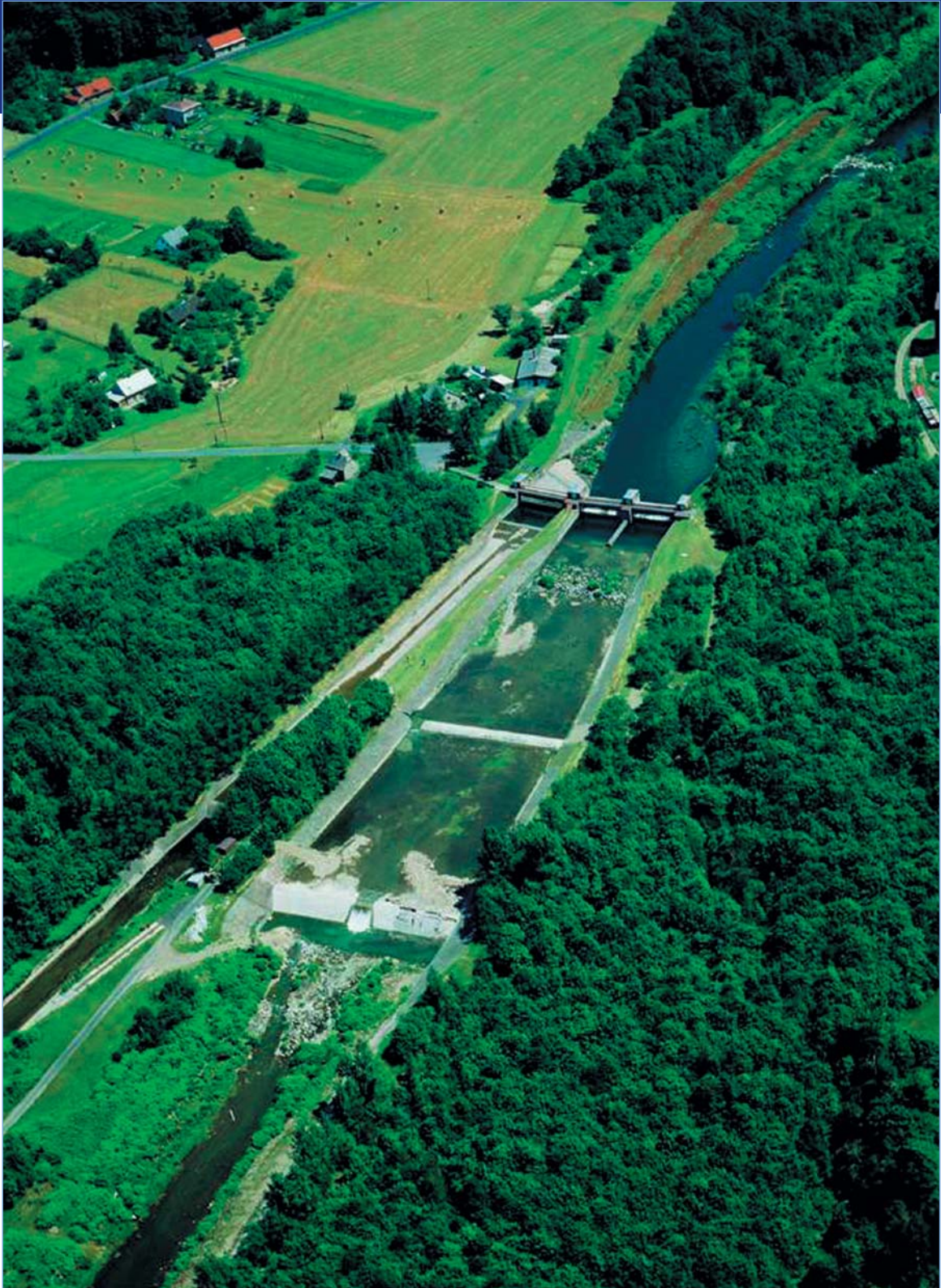
Weir at Morávka river - Odra river basin
