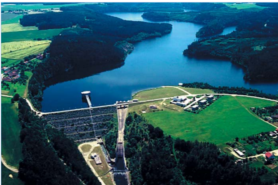
Řimov water reservoir - Vltava river basin
