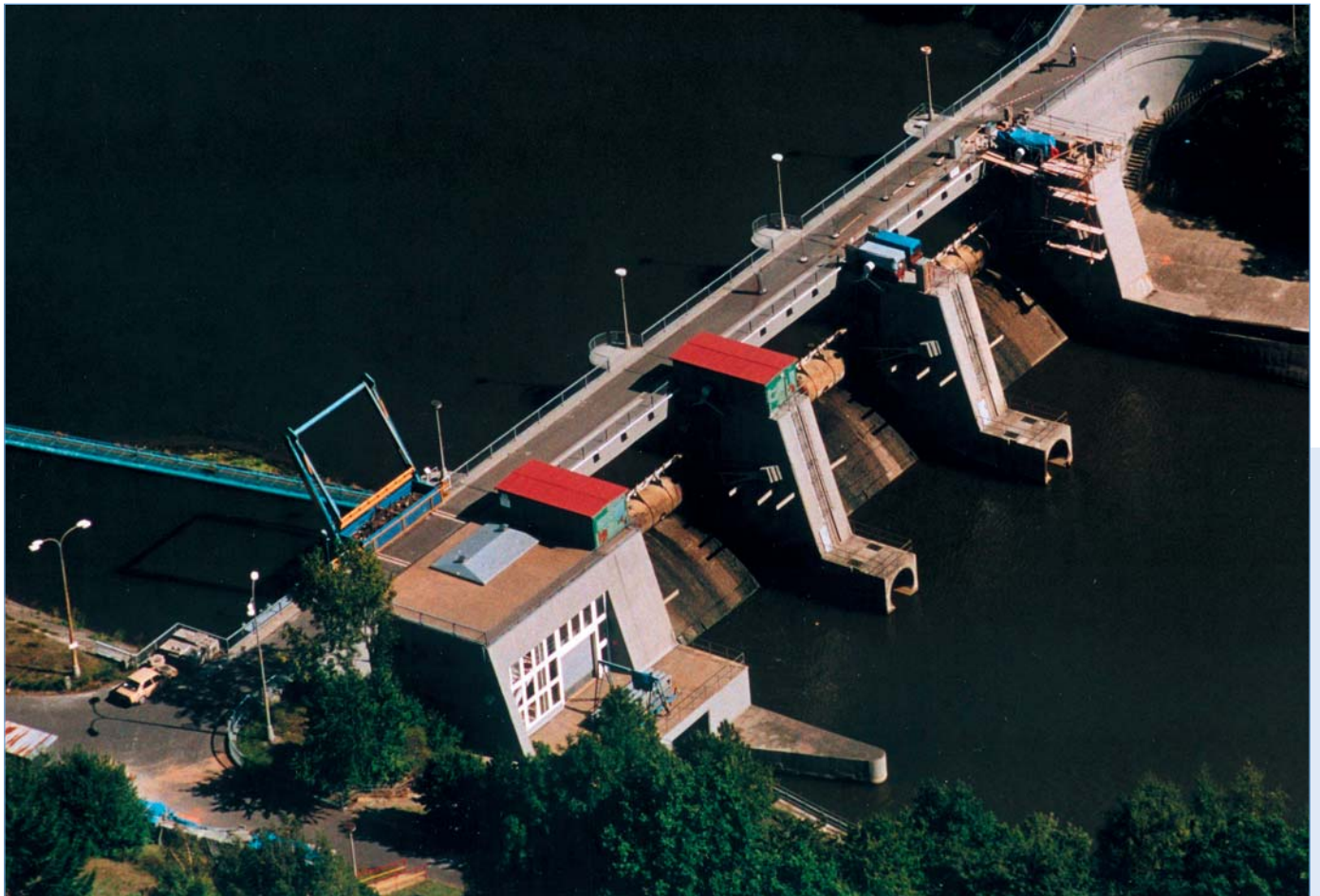
Kadaň water reservoir - Ohře river basin
