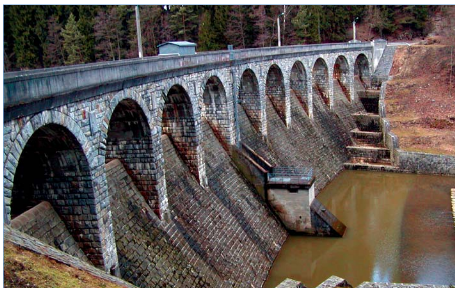
Sedlice water reservoir - Vltava river basin
