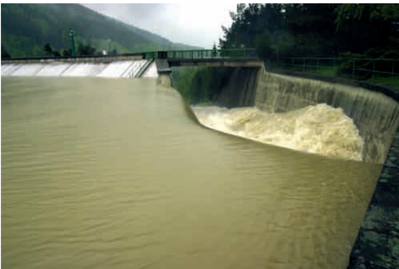
Safety spillway during flood peak in May 2010, hydraulic structure Morávka
