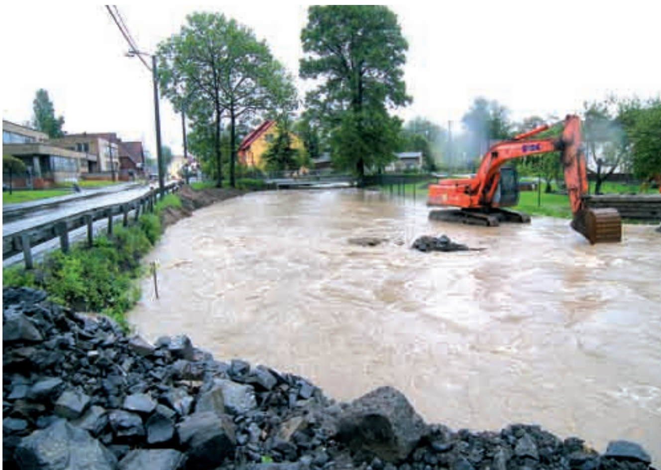
The Porubka River - torrent regulation after flood in 2010 in Ostrava-Svinov
