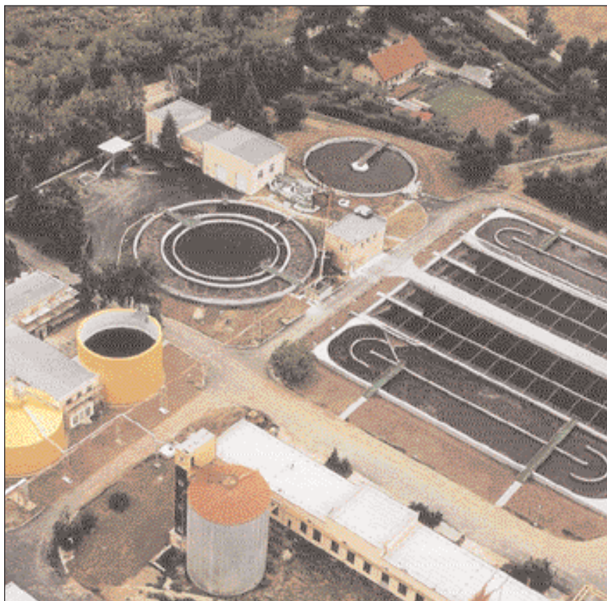
WWTP Kralupy nad Vltavou
