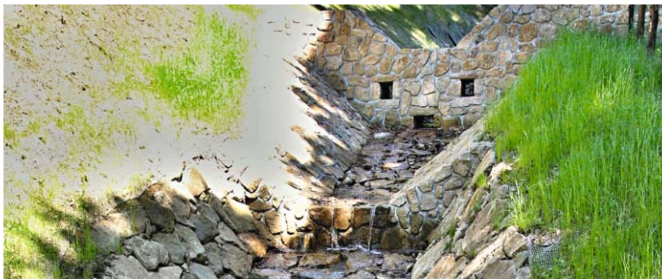
The Stream Bouřlivý, Mikulov – reconstruction of the streambed (source: Ohře River Basin, s. e.)
