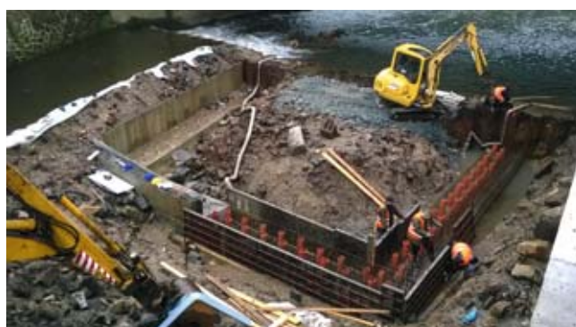
Fish crossing Hřensko – construction work (source: Ohře River Board, s. e.)
