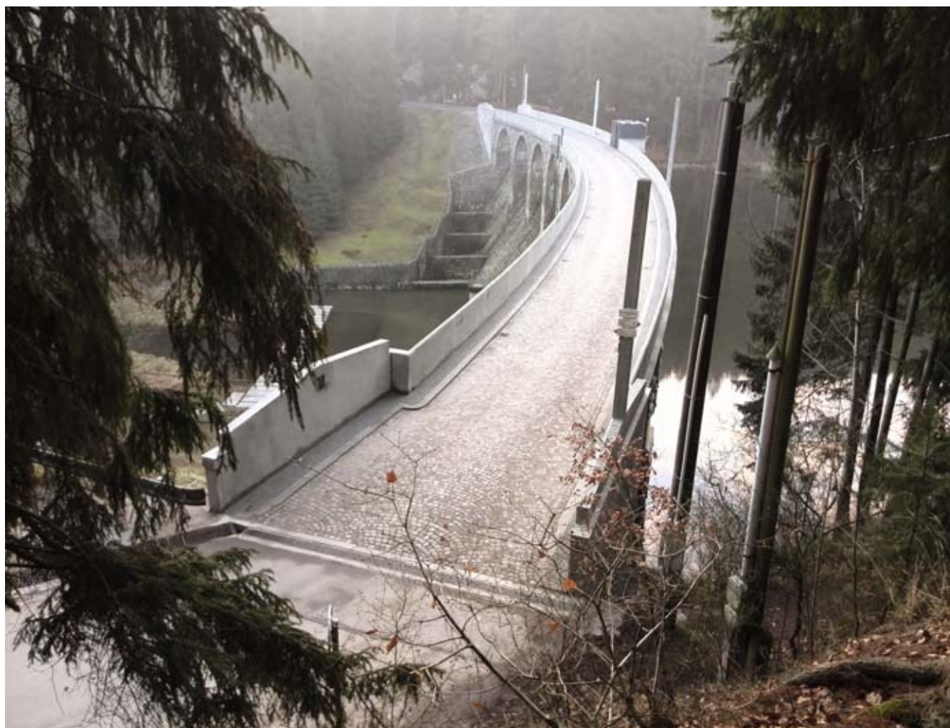
Water reservoir Sedlice – reconstruction of the crown and the upstream face of the dam (author: Jiří Kahánek)
