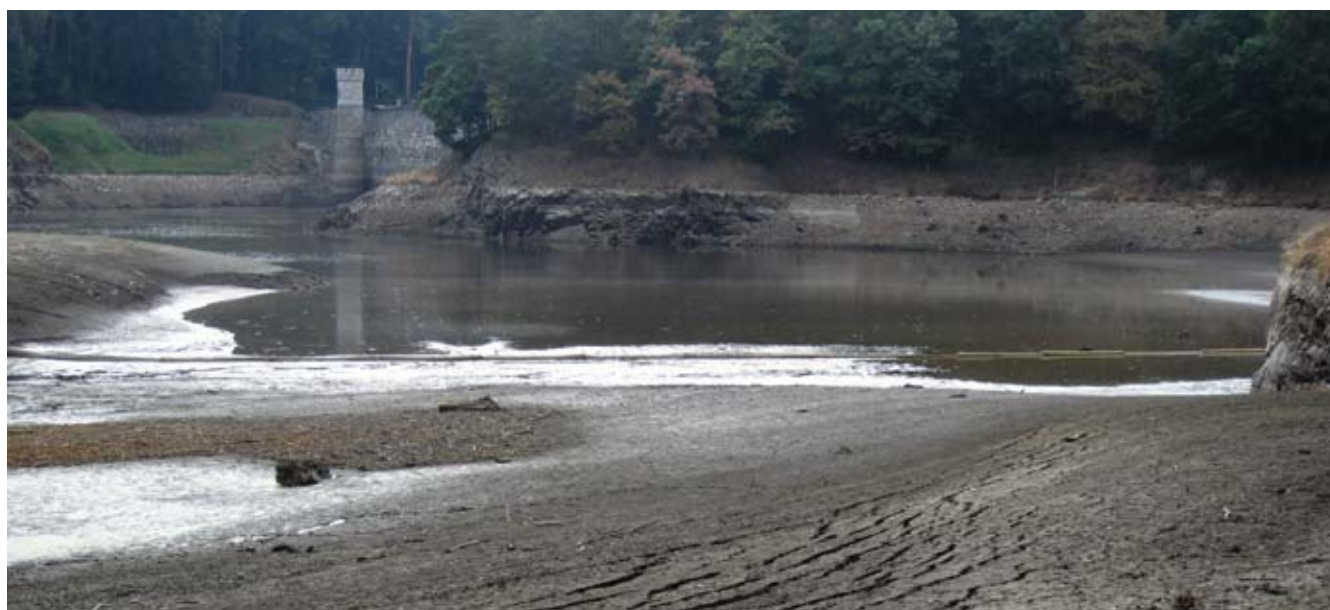
Water reservoir Pařížov, drought (source: Elbe River Board, s. e.)
