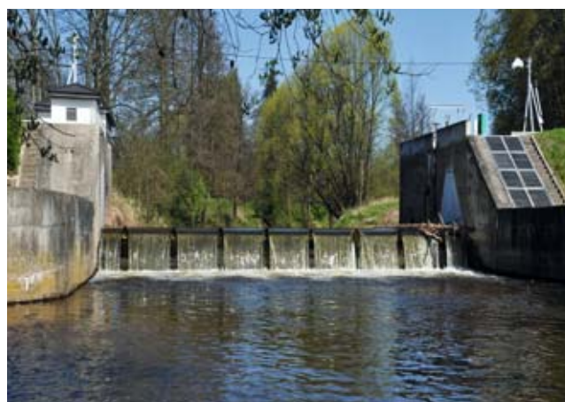
The weir on the Úpa River in Zlín (source: Elbe River Board, s. e.)
