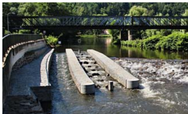
Fish crossing Loket – after implementation (source: Ohře River Board, s. e.)
