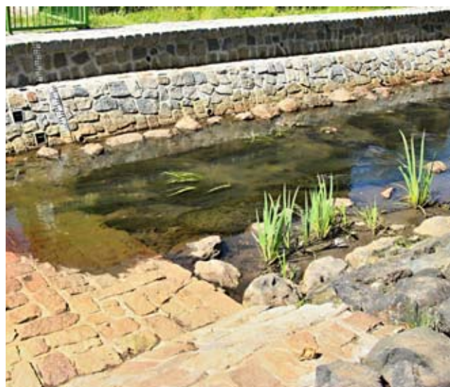
Revitalization of the Bouřlivec stream – Lahošť (source: Ohře River Board, s. e.)
