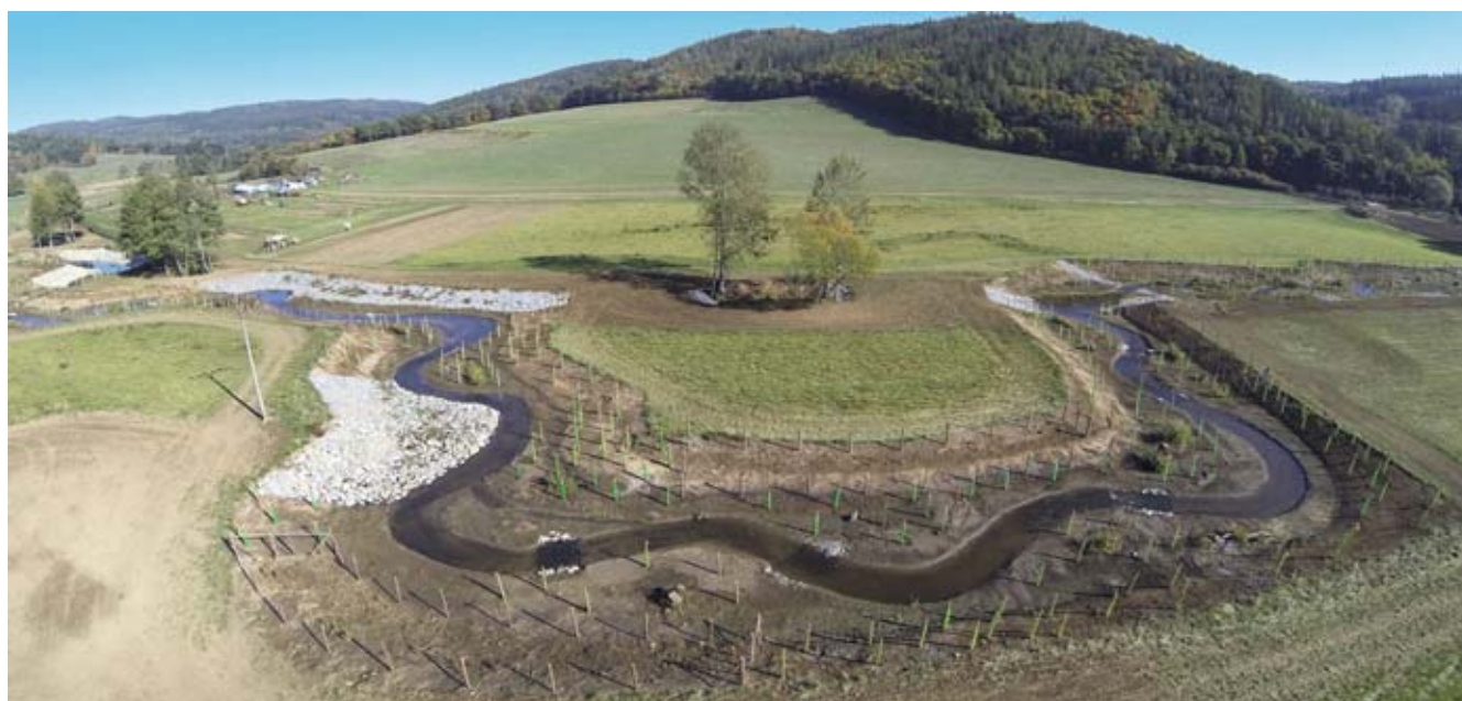
Revitalization of the watercourse Loděnice, Nenačovice (author: Aerodata, Ltd.)
