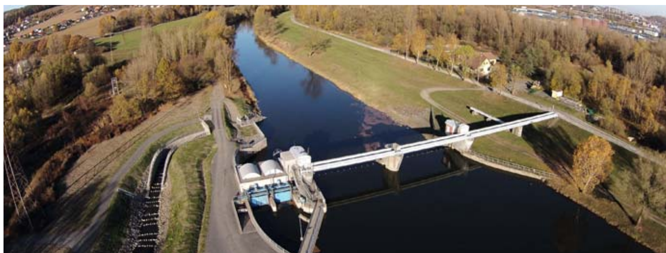
The weir Lhotka (source: Oder River Board, s. e.)
