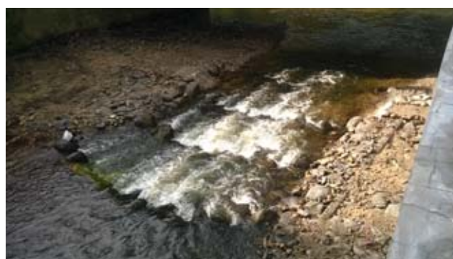
Fish crossing Hřensko – after implementation (source: Ohře River Board, s. e.)
