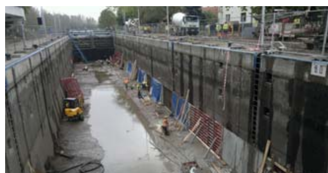
Repairing of the locks Brandýs nad Labem (source: Elbe River Board, s. e.)
