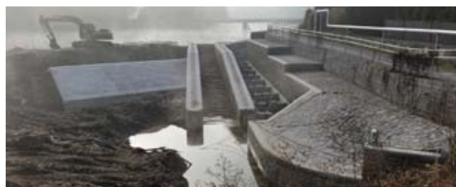
Reconstruction of the weir Černošice, the Berounka River – part of a work fish crossing (author: Jan Šimůnek)
