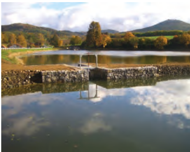
The Bilka Small Water Reservoir after renovation (author: Josef Vitek)
