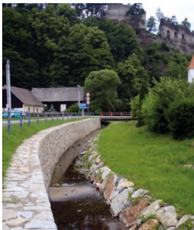
Flood protection, the Křeslice Stream, 0.000–1.002 km, 2009 (source: Forests of the Czech Republic, s. e.)
