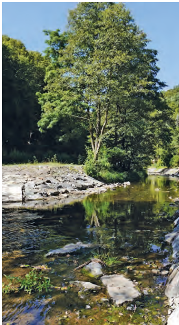
The Kocába River, Masečín, renovation of the river basin bulwark (author: Šárka Hermanová)
