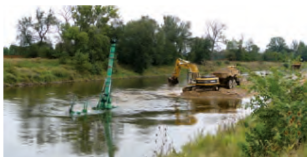
The Vltava River at Vraňany, removal of sediments and repair of the bulwark (author: Richard Pawinger)
