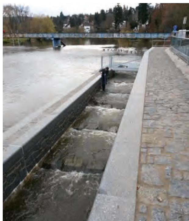
Černošice, a fish pass (source: Vltava River Board, s. e.)
