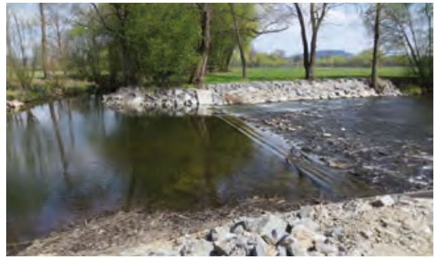
The Úhlava River, renovation of the Poborovice Weir (author: Miloslav Křen)
