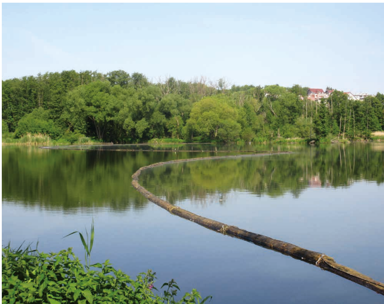
The Podhradský Pond – newly installed an ible wall, May 2017 (source: Morava River Board, s. e.)
