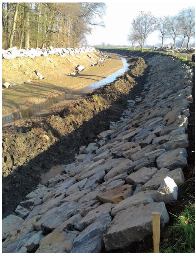
Bat'a Canal – Vnorovy, Renovation of the bank protections, autumn 2017 (source: Morava River Board, s. e.)
