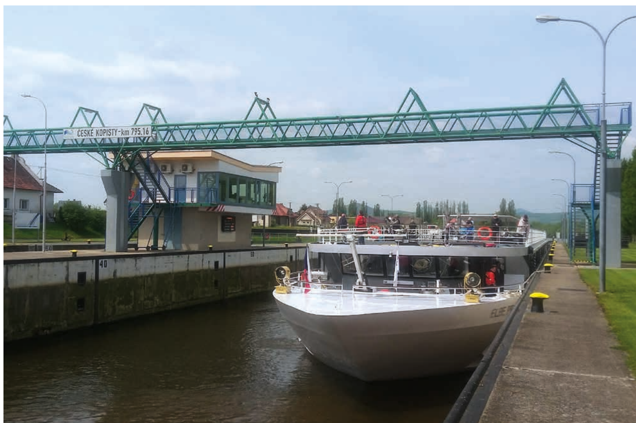
The Big Lock Chamber of the České Kopisty Dam (source: Elbe River Board, s. e.)
