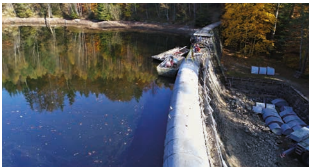
The Naděje Dam – Renovation of Safety Spillway Crest (source: Ohře River Board, s. e.)
