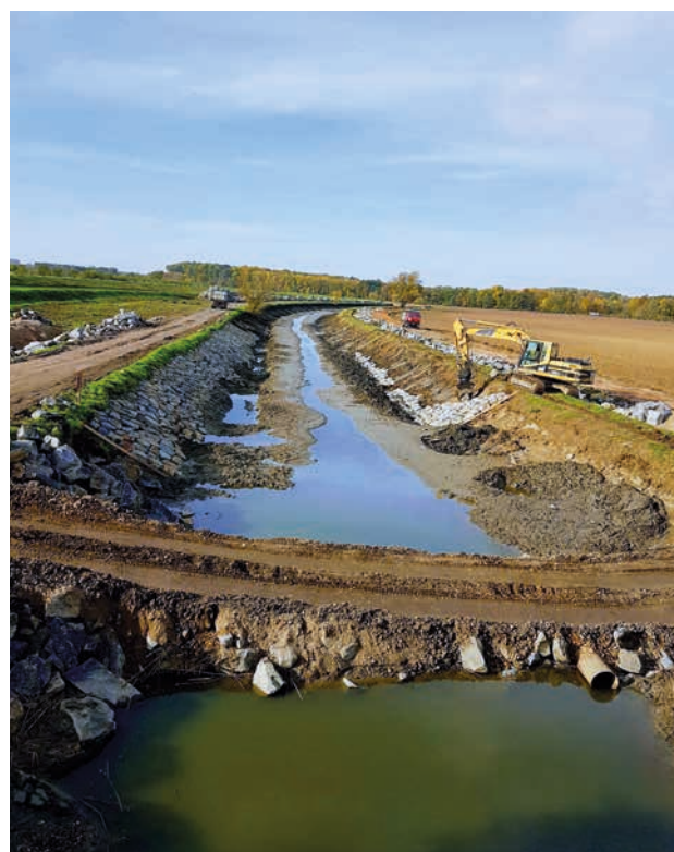
Renovation of the bank protections and banks of Bat'a canal, Vnorovy, October 2017 (source: Morava River Board, s. e.)
