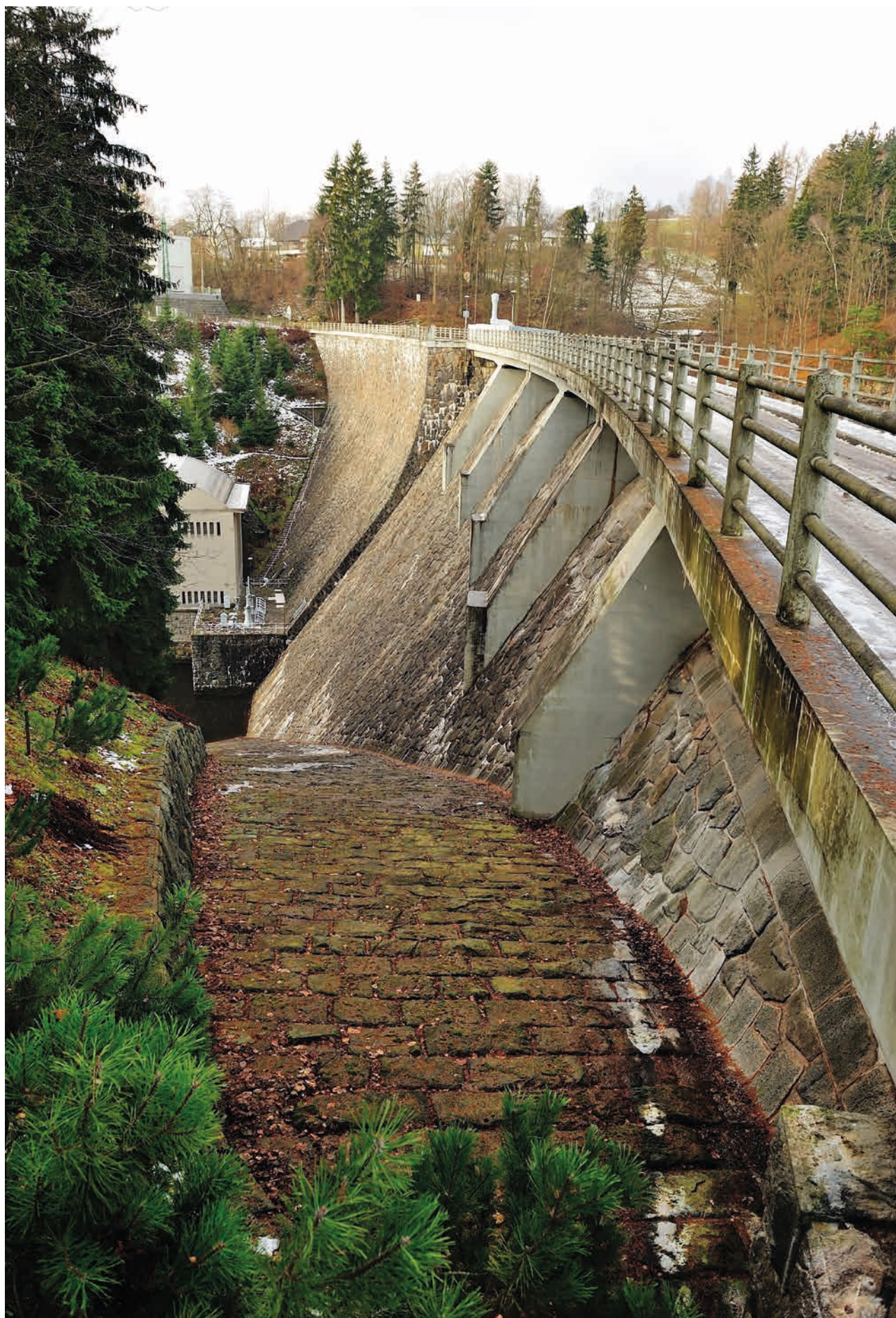
The Pastviny Dam (source: Elbe River Board, s. e.)
