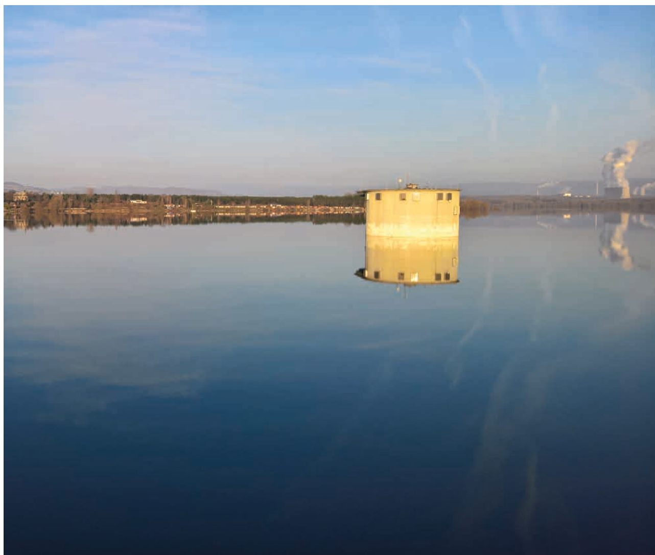
The Nechranice Dam (source: Ohře River Board, s. e.)
