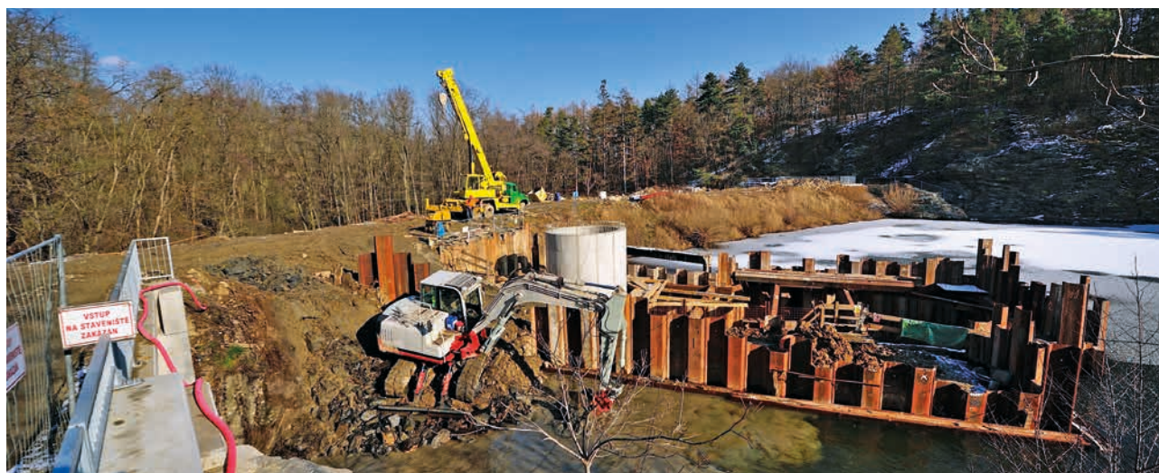
The Pond Velký rybník – restoration of bottom drains (source: Elbe River Board, s. e.)
