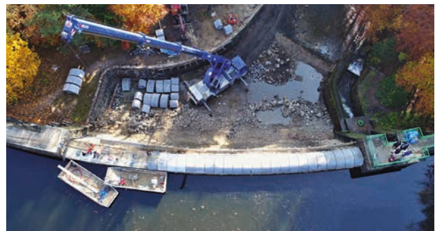
The Naděje Dam – Renovation of Safety Spillway Crest (source: Ohře River Board, s. e.)
