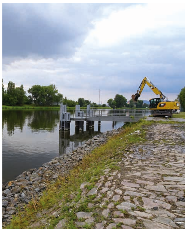
The Riprap Treating, Litoměřice (source: Elbe River Board, s. e.)
