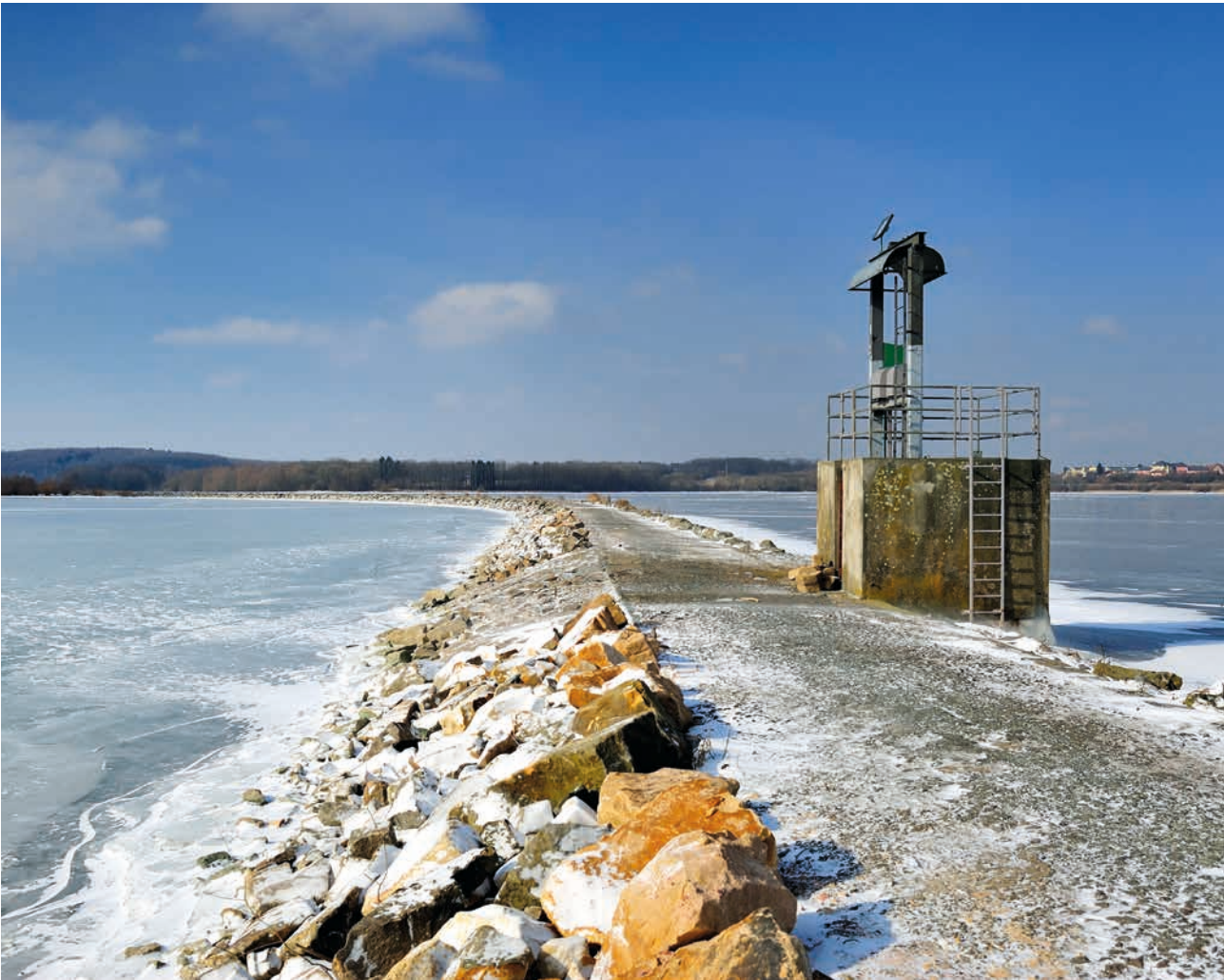
The Rozkoš Dam (source: Elbe River Board, s. e.)
