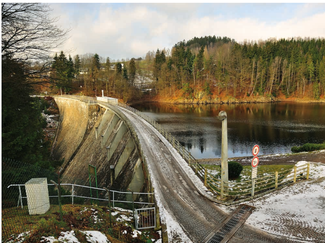
The Pastviny Dam (source: Elbe River Board, s. e.)
