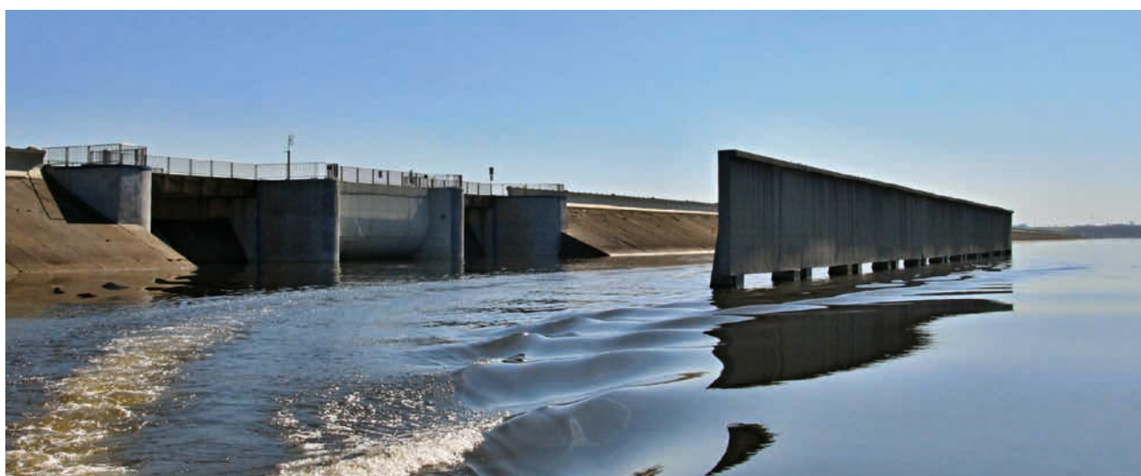
The Nechanice Dam (source: Ohře River Board, s. e.)
