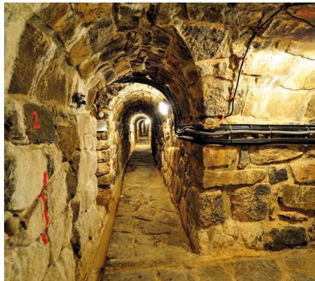
The Tunnel in the Levee of the Pastviny Dam (source: Elbe River Board, s. e.)
