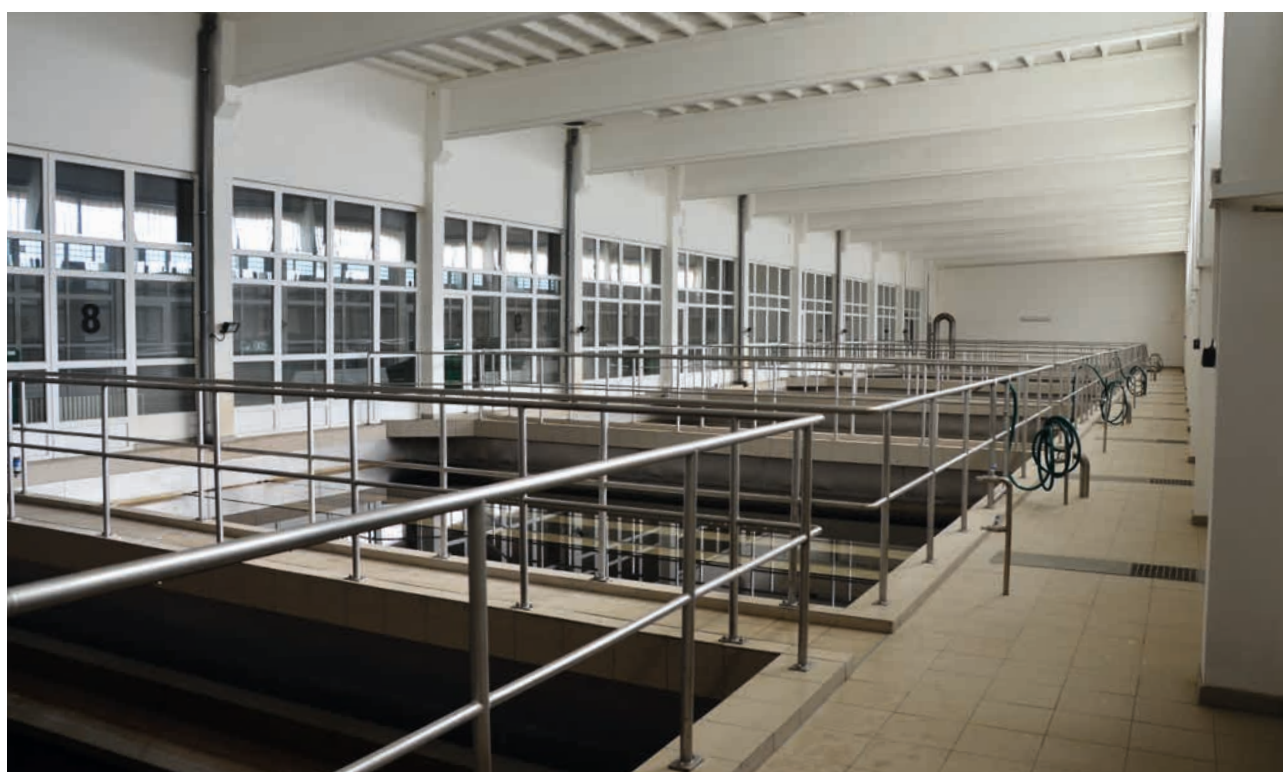
Water Treatment Plant Káraný (author: Martin Mareš)
