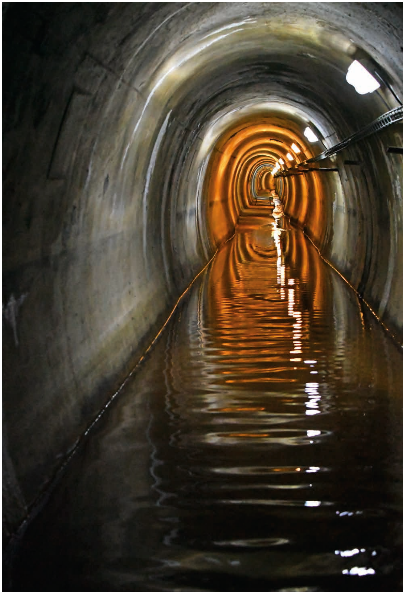
Drainage Chanel, The Josefův Důl Dam (source: Elbe River Board, s. e.)
