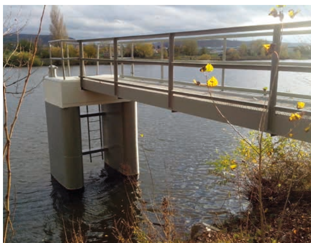
The Berounka River – Repairing of Dolphin (source: Vltava River Board, s. e.)
