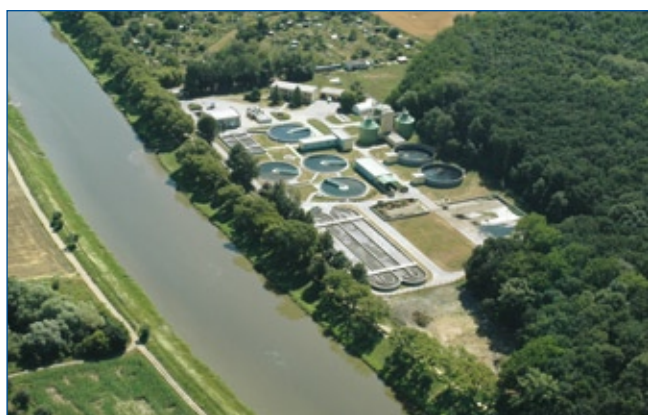
The Morava River– waste water treatment plant Uherské Hradiště
