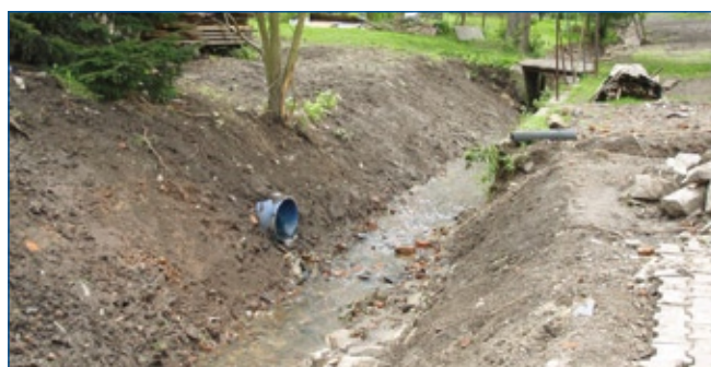
Remedying of flood damage to the Česká Kamenice River
