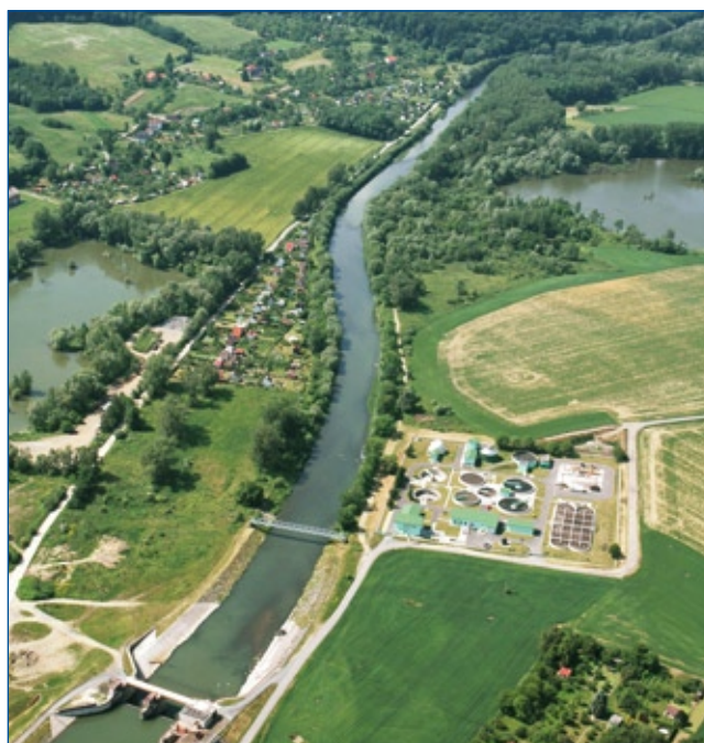
The Bečva River – waste water treatment plant Hranice na Moravě
