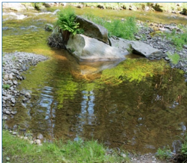
The Fishpassing facilities on the Blanice River
