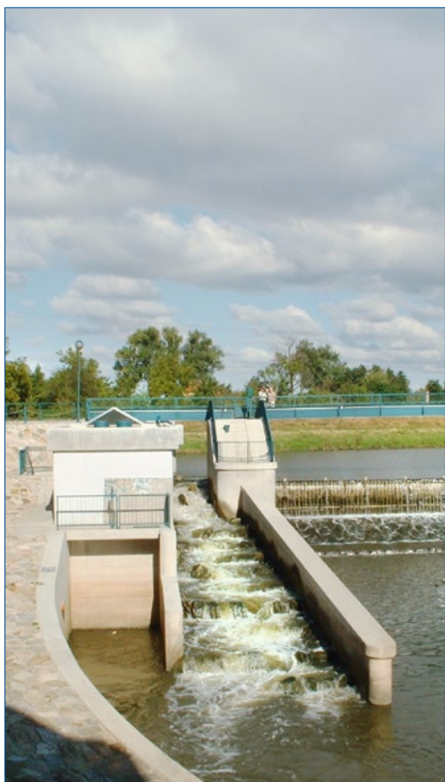
The Fishpassing facilities in Veselí
