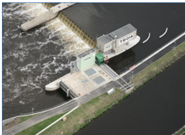
The Vltava River – small hydroelectric power plants Troja
