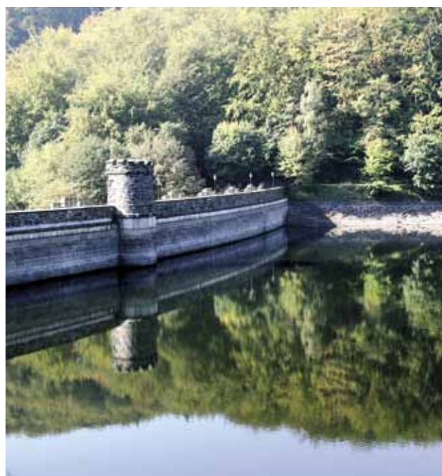
Hydraulic structure Kamenička
