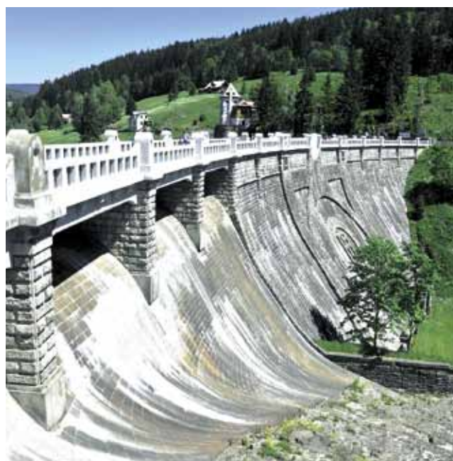
Hydraulic structure Labská, the Labe River
