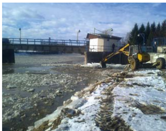
Weir in Osek - removing ice at the inlet sluice
