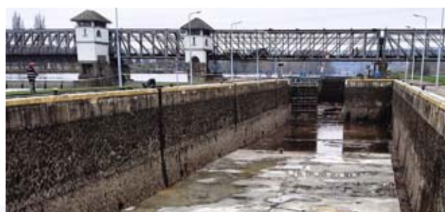
Mířejovice hydraulic structure, reconstruction of the lock bottom
