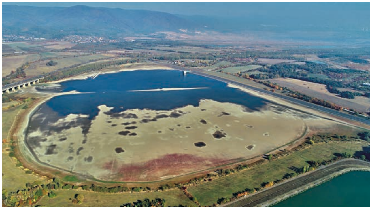
The Újezd Dam, up The July 2018, down The October 2018 (source: Ohře River Board, s. e.)
