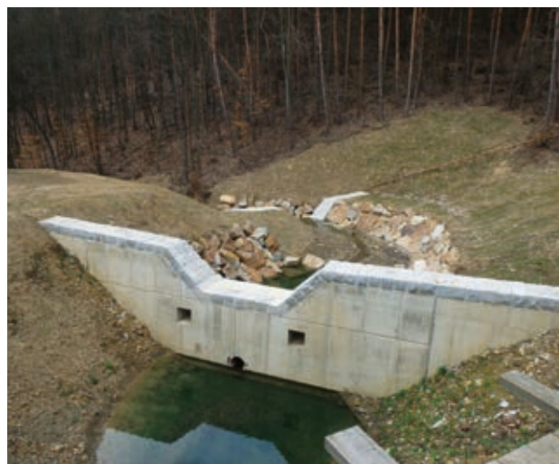
Right Bank Tributary of Kudlovický Stream (source: Forest of the Czech Republic, s. e.)
