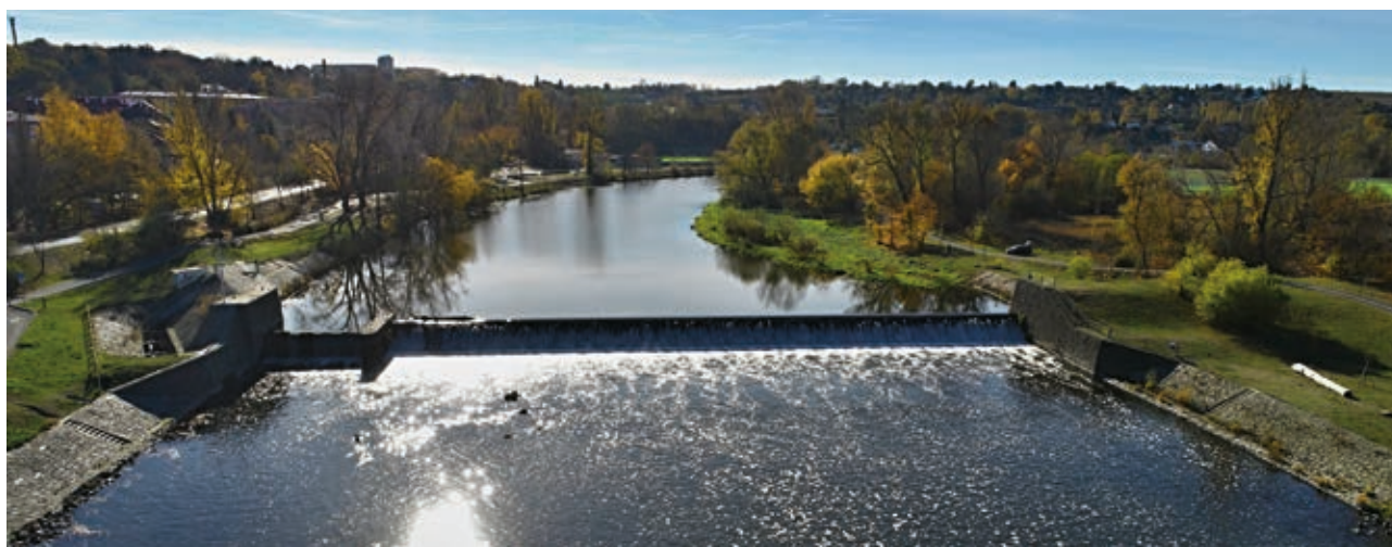
The Žatec Weir (source: Ohře River Board, s. e.)
