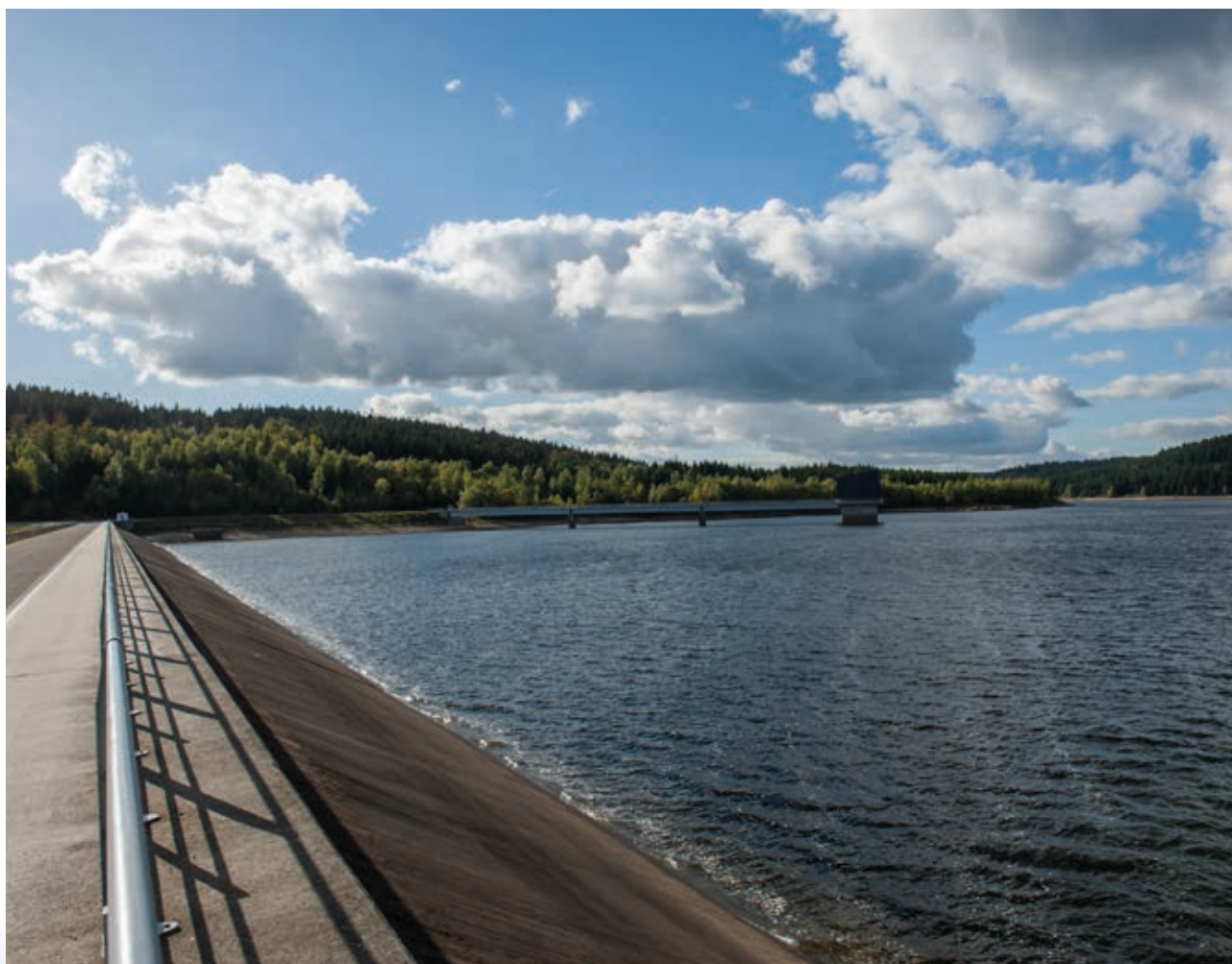
The Josefův Důl Dam (source: Elbe River Board, s. e.)
