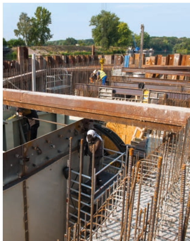
Construction of a Small Hydroelectric Power Plant Veletov (source: Elbe River Board, s. e.)
