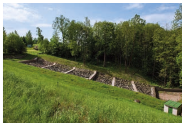
The Jahodnice Safety Spillway (source: Elbe River Board, s. e.)
