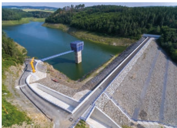
The Opatovice Dam, after the Reconstruction (source: Morava River Board, s. e.)
