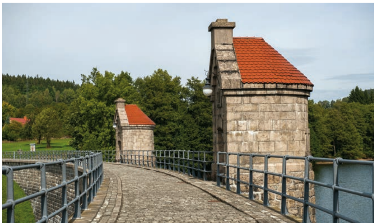
The Mlýnice Dam (source: Elbe River Board, s. e.)
