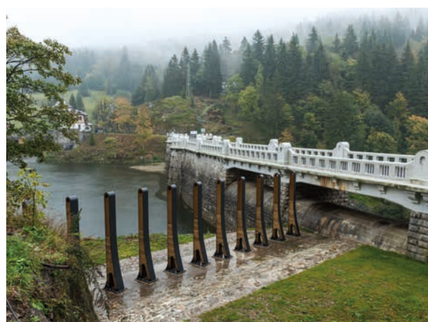
Dam at the Labská Water Reservoir (Source: Elbe River Board)
