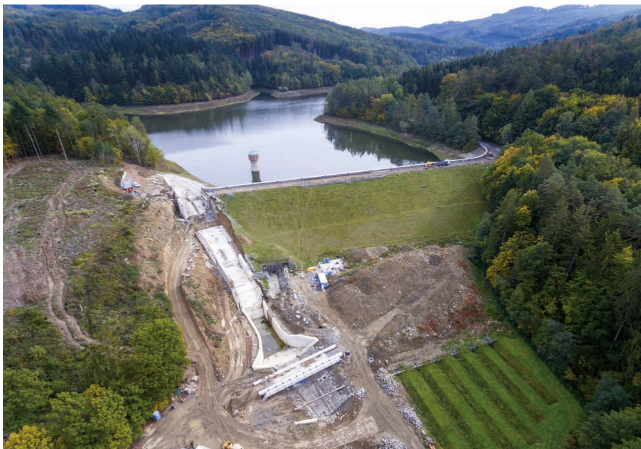
Reconstruction of the Koryčany Water Reservoir (Source: Morava River Board)
