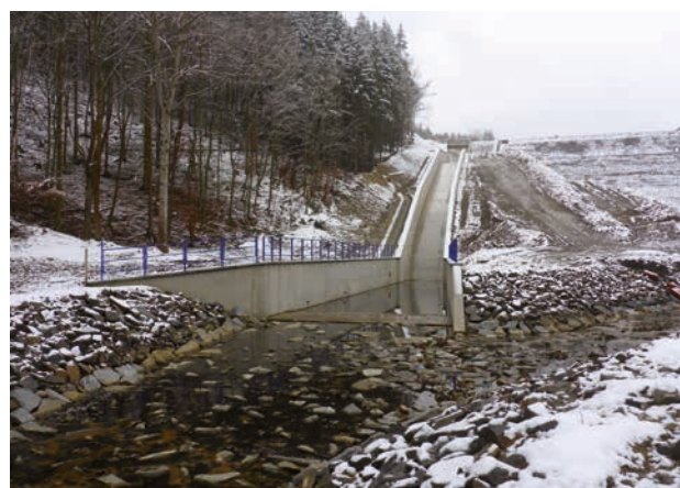
Completed chute at the Opatovice Water Reservoir (Source: Morava River Board)
