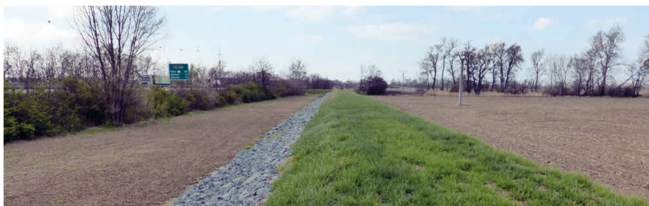
Flood protection of the town of Pohořelice: construction of 6,450 m of protective dams and walls (Source: Morava River Board)
