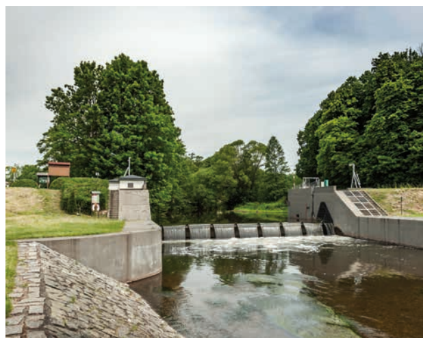
Zlích Weir (Source: Elbe River Board)
