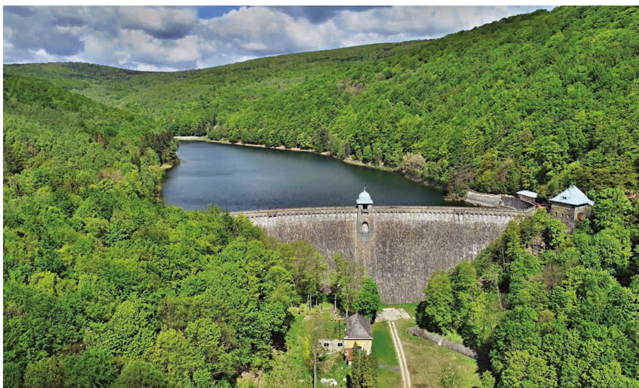
Janov Water Reservoir, May 2020 (Source: Ohře River Board)
