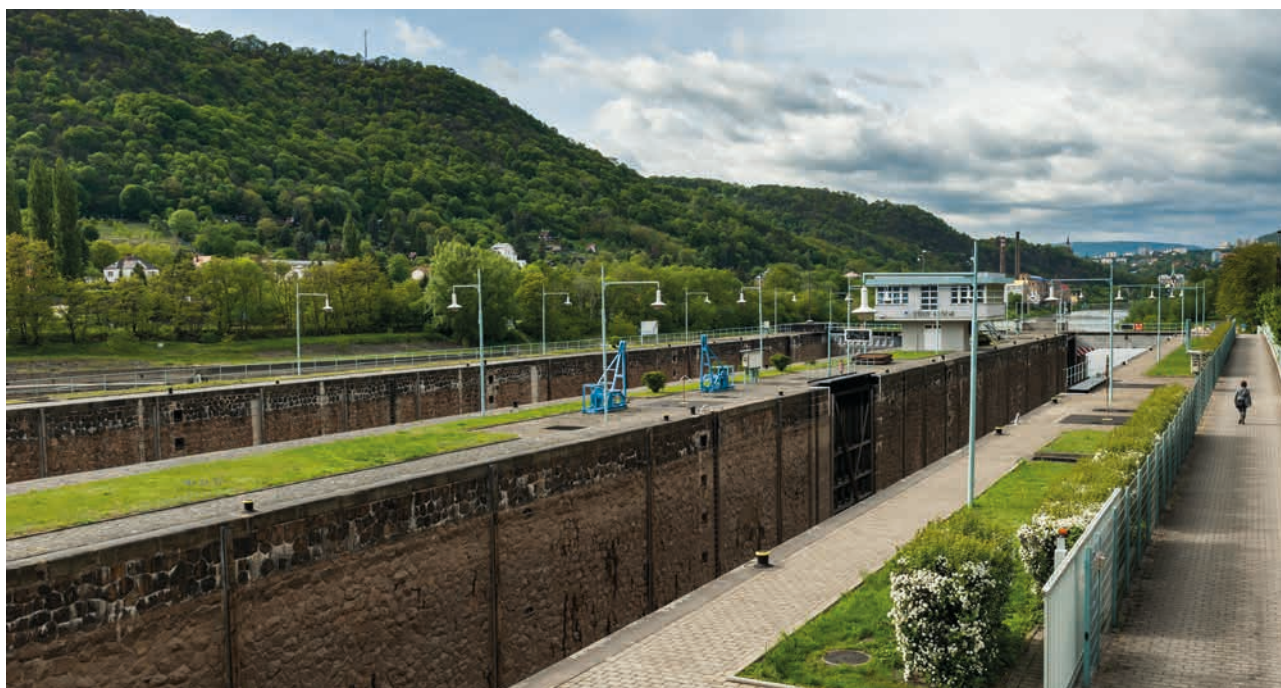
Střekov lock chambers (Source: Elbe River Board)
