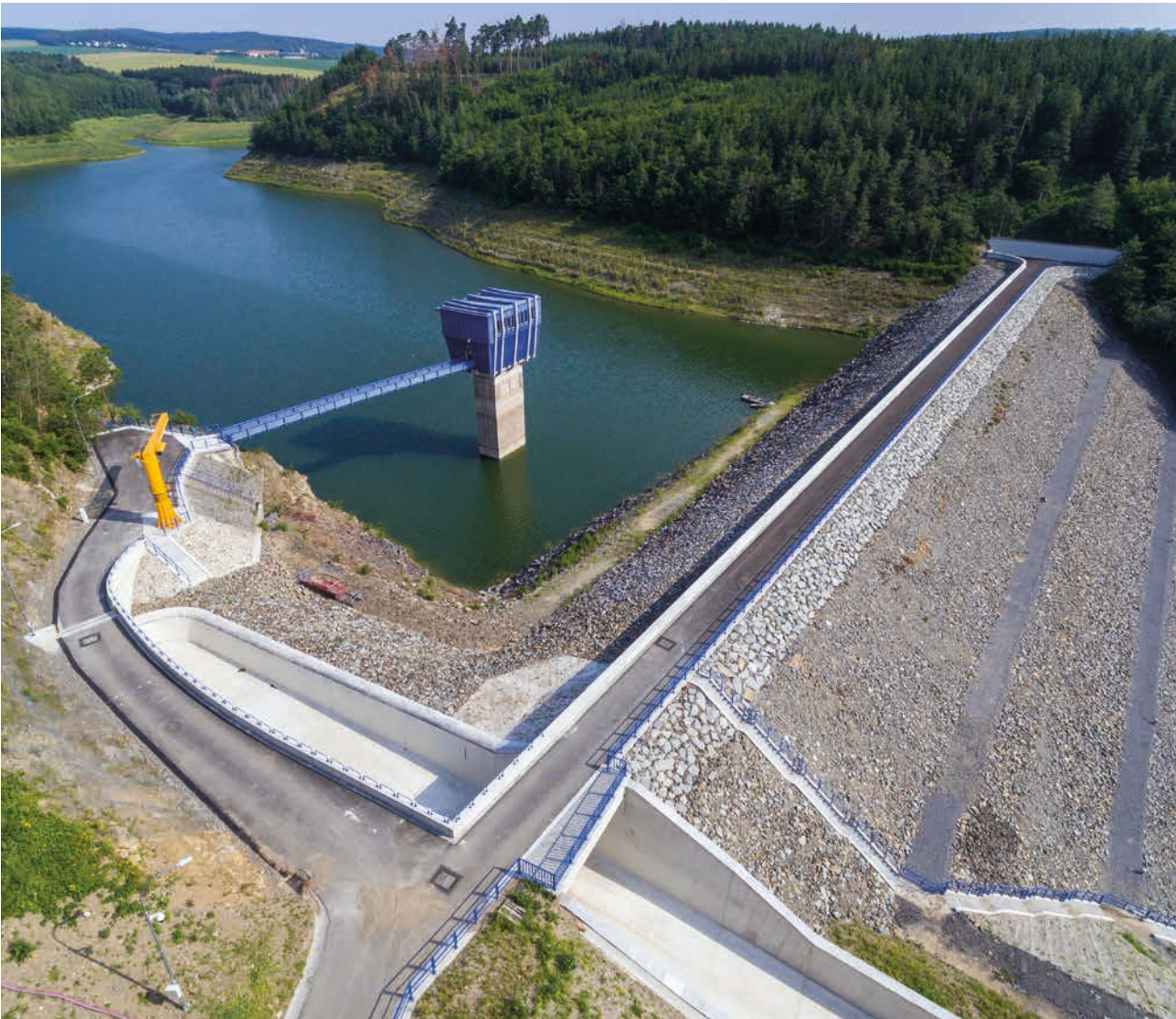
Opatovice Water Reservoir after reconstruction (Source: Morava River Board)
