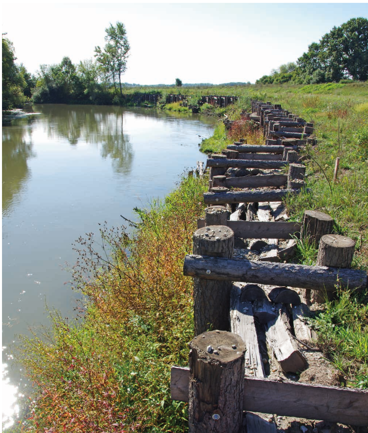
Cross-border project of reintegrating weaned shoulders of the Dyje River: a shoulder of the Dyje River reinforced with willow fences (Source: Morava River Board)
