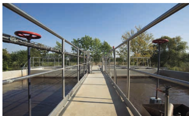
WWTP Prosiměřice reconstruction and intensification (Source: MoE)
