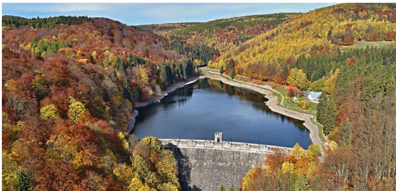
Kamenička Water Reservoir (Source: Ohře River Board)
