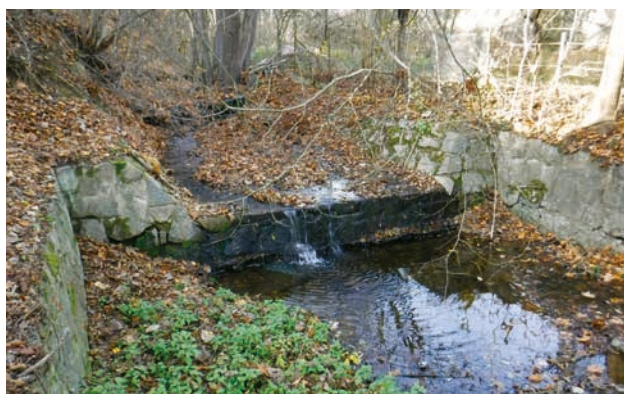
Nihošovický Stream, Nihošovice – regulation before repair (Source: Vltava River Board)
