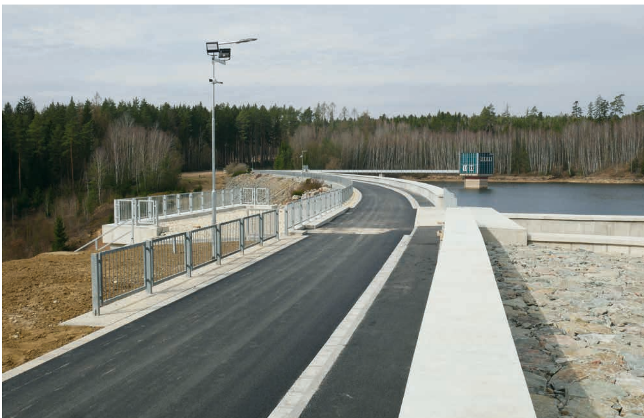
Dam crest after reconstruction at the Boskovice Water Reservoir (Source: Morava River Board)
