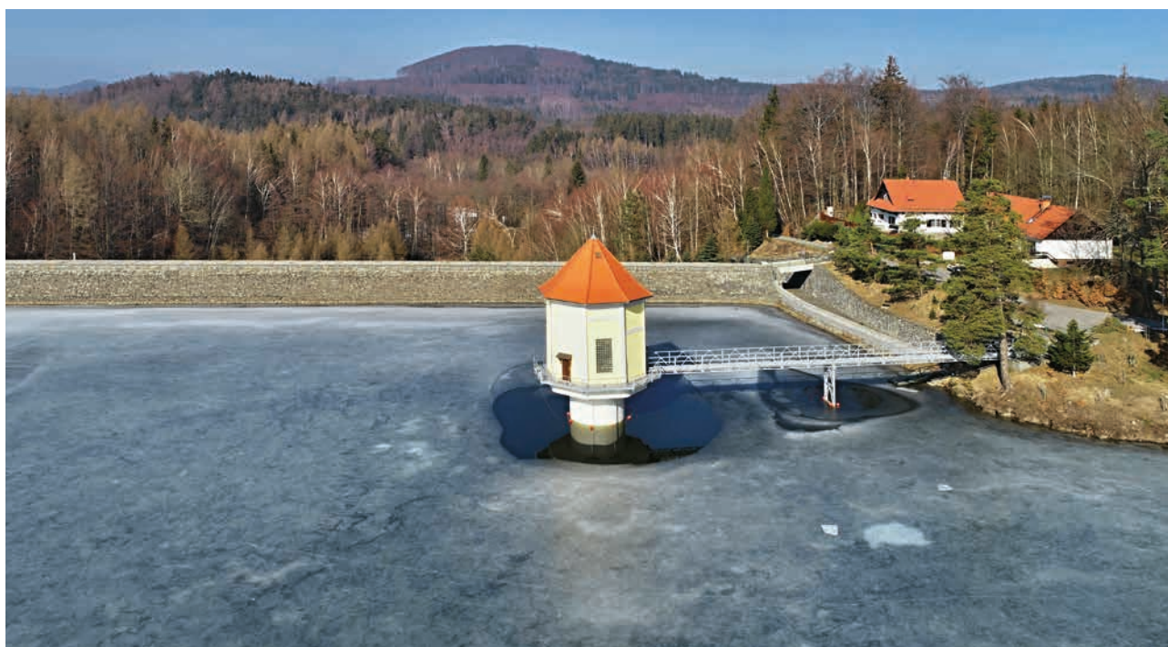
Chřibská Water Reservoir, February 2020 (Source: Ohře River Board)
