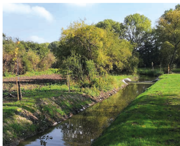
New retention damming in the Dunávka Stream ensure constant presence of water and favourable conditions for water organisms (Source: Morava River Board)
