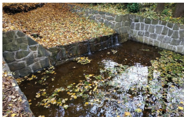
Nihošovický Stream, Nihošovice – regulation after repair (Source: Vltava River Board)
