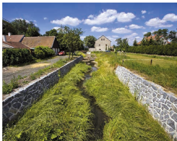
Flood protection of the municipality of Žiželice (Source: MoE)
