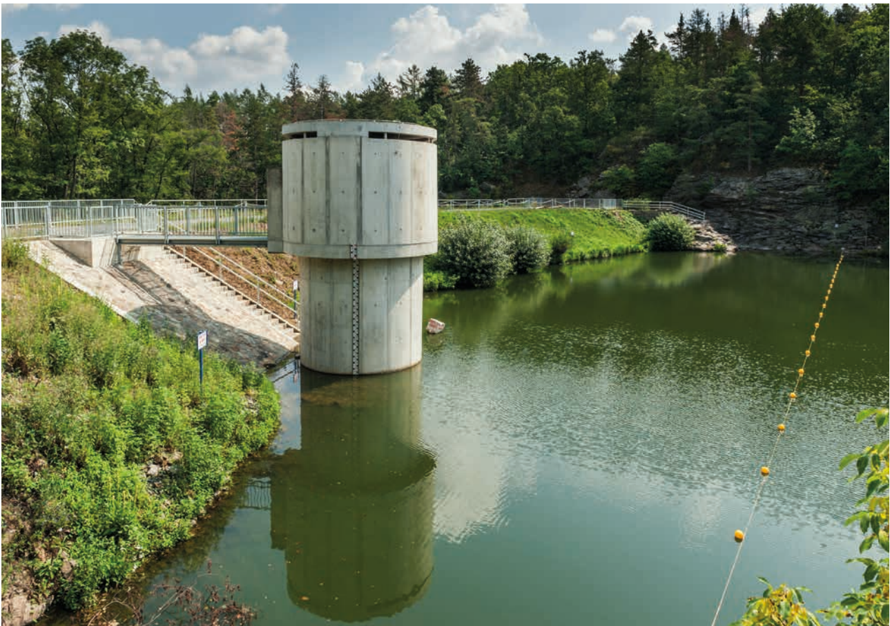
Large Pond (Source: Elbe River Board)
