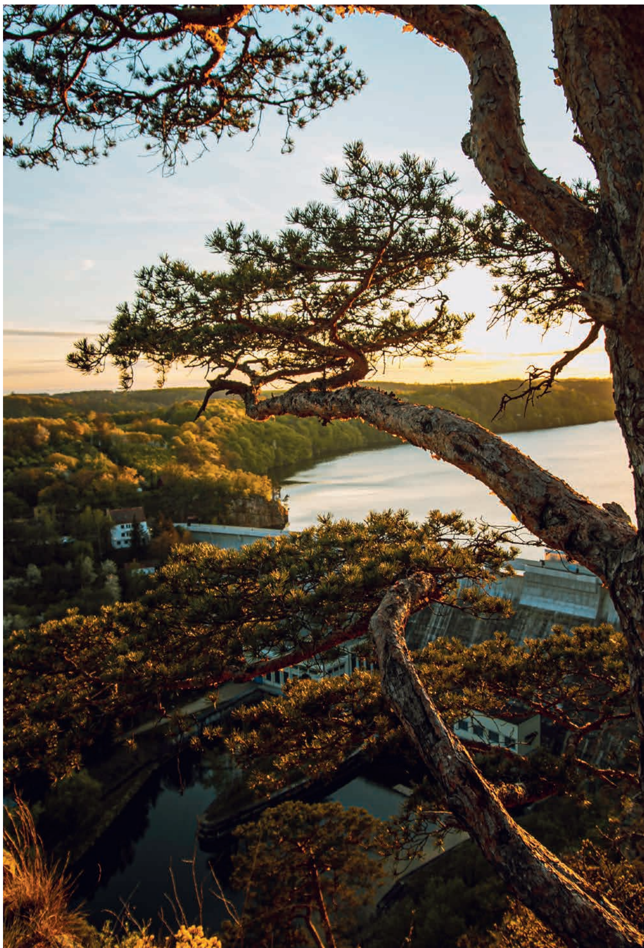
View Through the Pines, May 2021, The Vranov nad Dyji Dam (author: Grund Petr)
