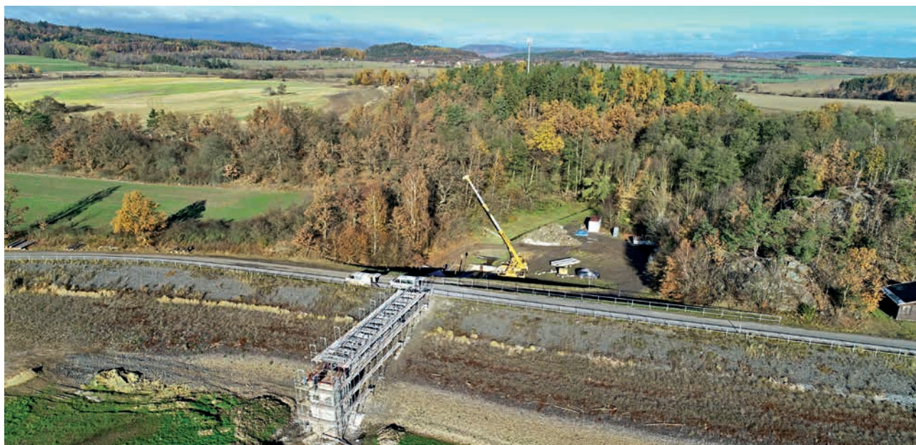
The Blatno construction (source: Ohře River Board, s.e.)
