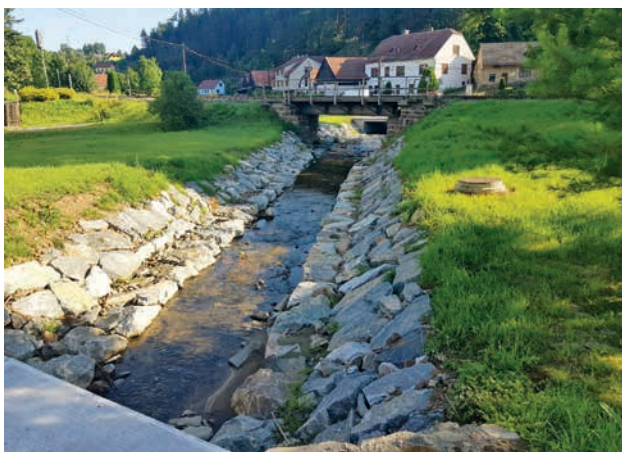
Increasing the capacity of the Rožinka stream in the urban area of the village of Rožná in Žďársko (source: Forest of the Czech Republic, s.e.)
