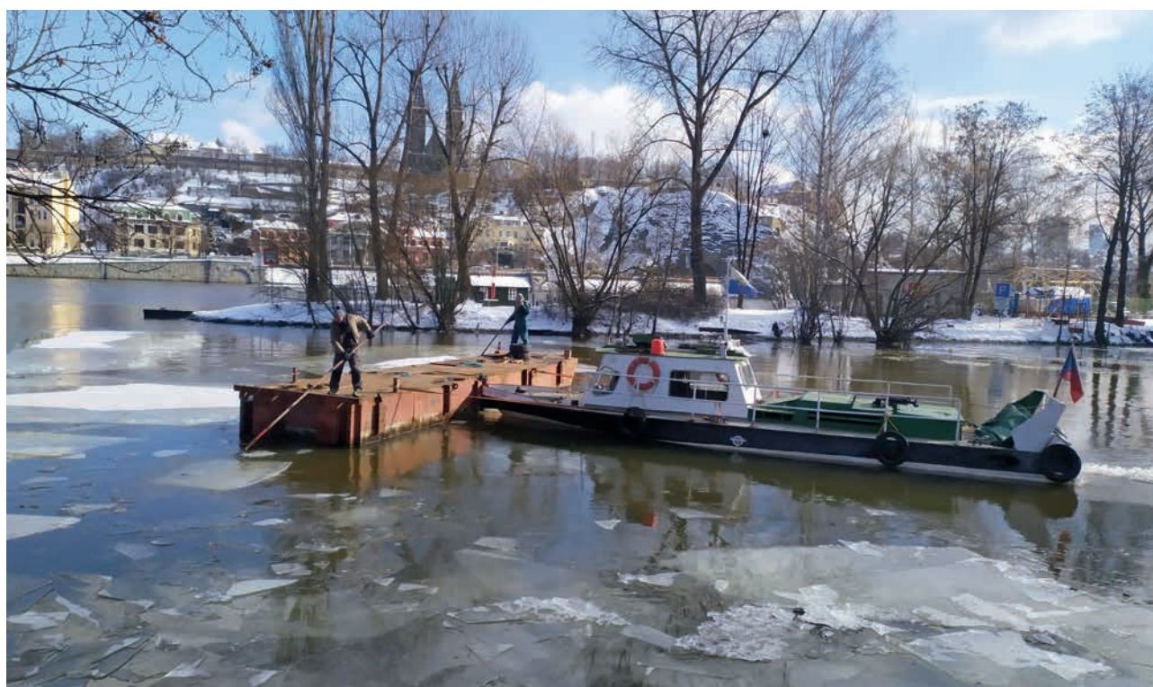
The Vltava stream, the Port of Prague Smíchov – demolition of the ice mainland (source: Vltava River Board, s.e.)
