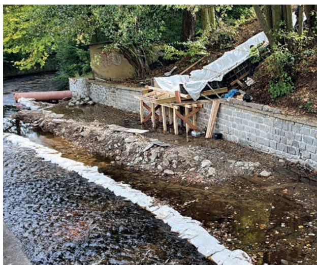
The Construction on the Chomutovka Stream (source: Ohře River Board, s.e.)
