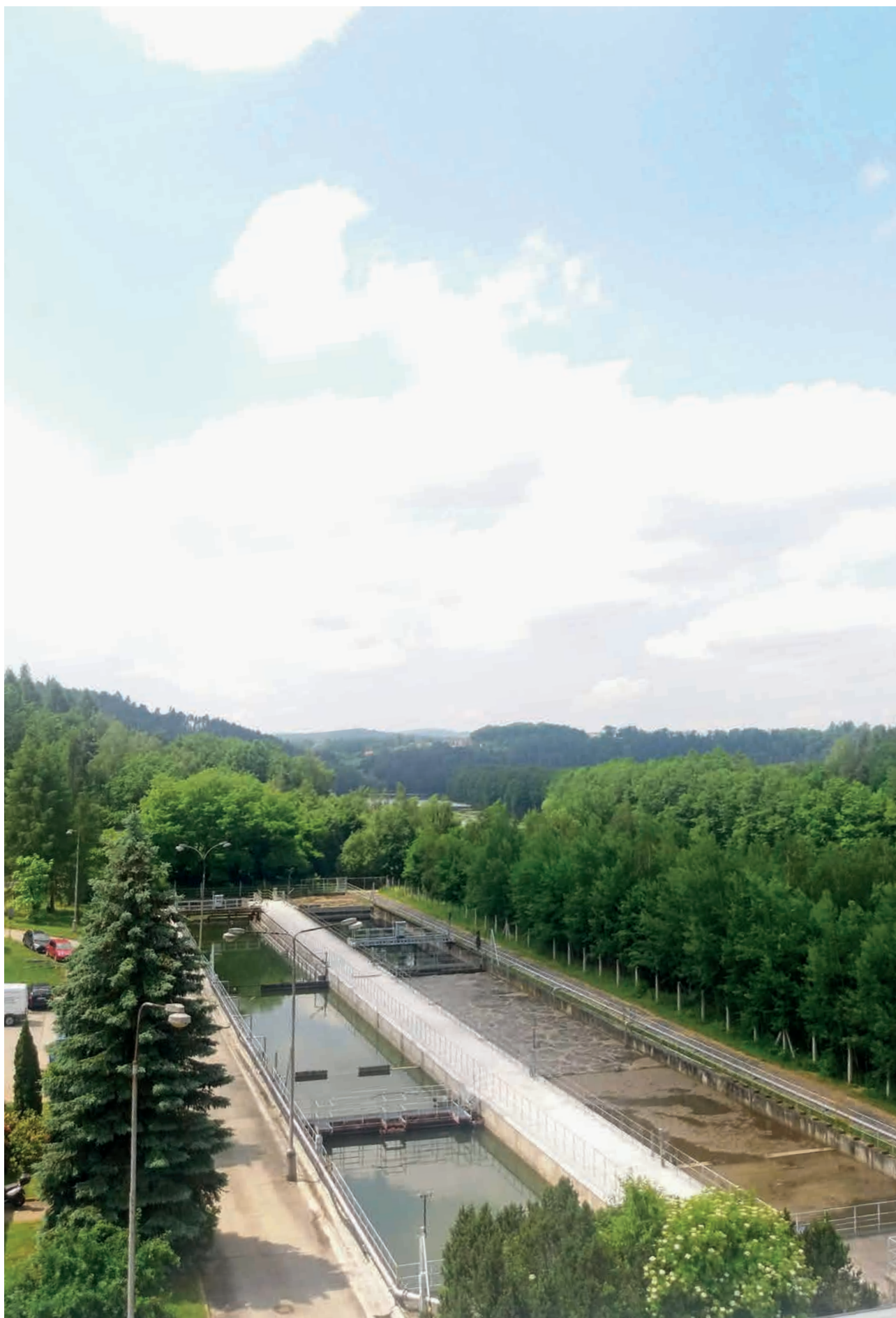
The Wastewater Treatment Plant, Týn nad Vltavou (author: Hubalová Petra)
