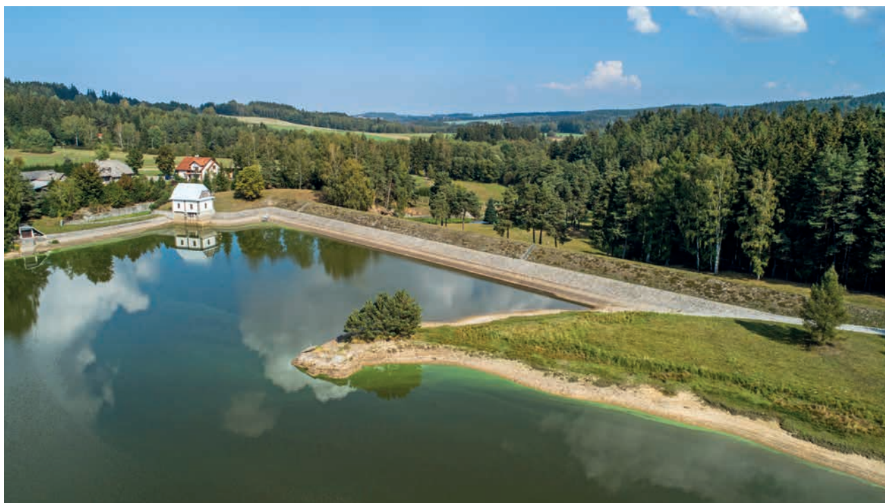
The Hamry Dam (source: Elbe River Board, s.e.)
