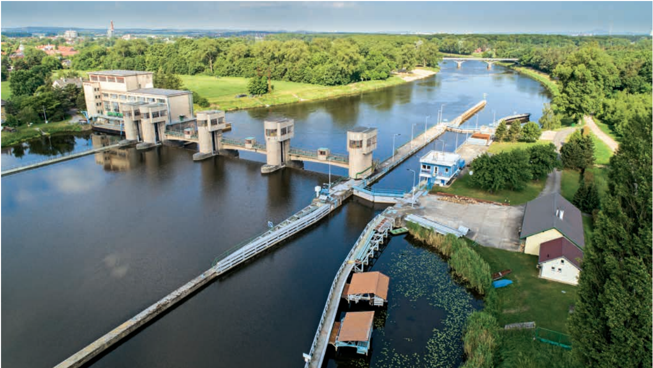
Kostelec lock on the Elbe waterway (source: Elbe River Board, s. e.)
