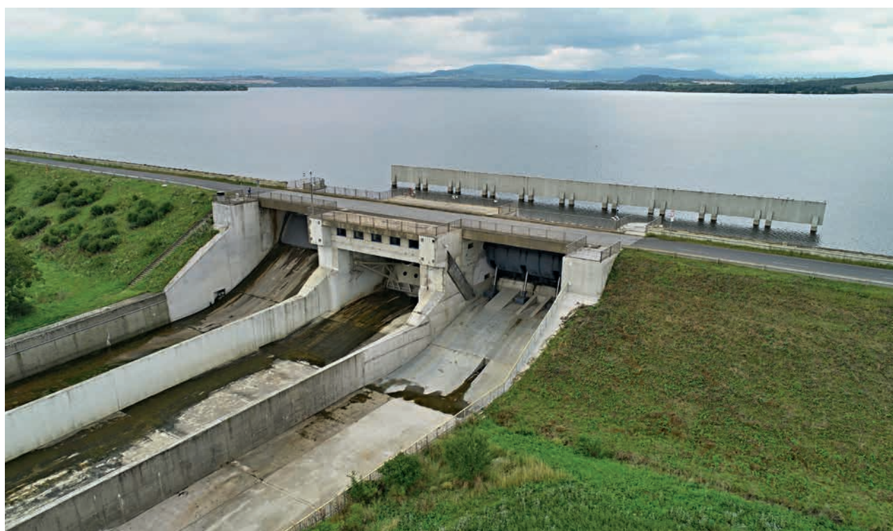
The Nechanice Dam (source: Ohře River Board, s.e.)
