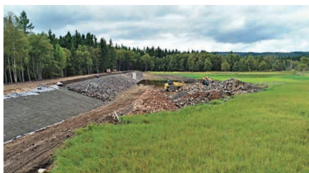
The Old Pond, the construction (source: Ohře River Board, s.e.)
