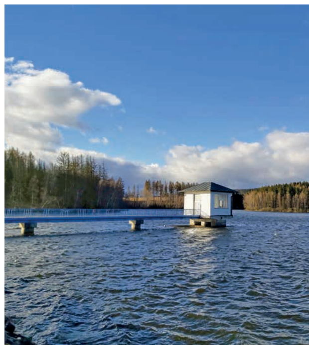
The Hubenov Dam, the full status (author: Kučerová Jana)
