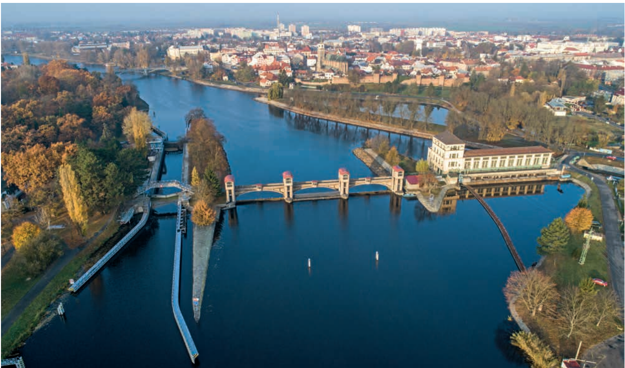
Nymburk lock on the Elbe waterway (source: Elbe River Board, s.e.)
