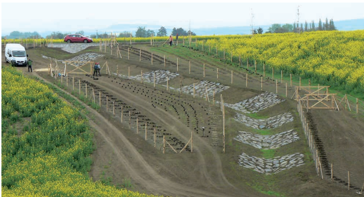
Construction of anti-erosion and flood protection measures in the cadastral area Hruška (source: State Land Office)
