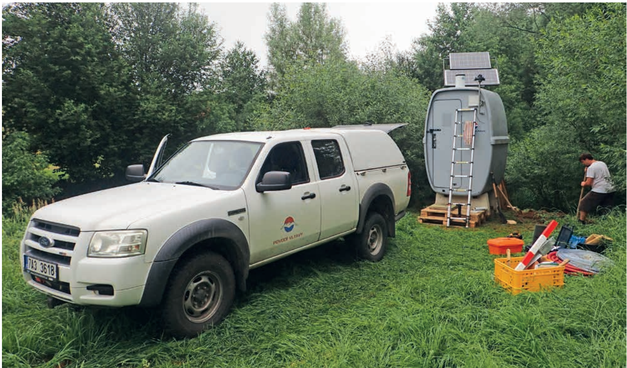
Sampler installation, Hořepník (source: Vltava River Board, s.e.)
