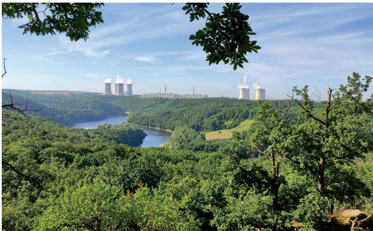
Cooling water pumping station for the Dukovany Nuclear Power Plant, July 2021, The Mohelno Dam (author: Pavlíková Eliška)
