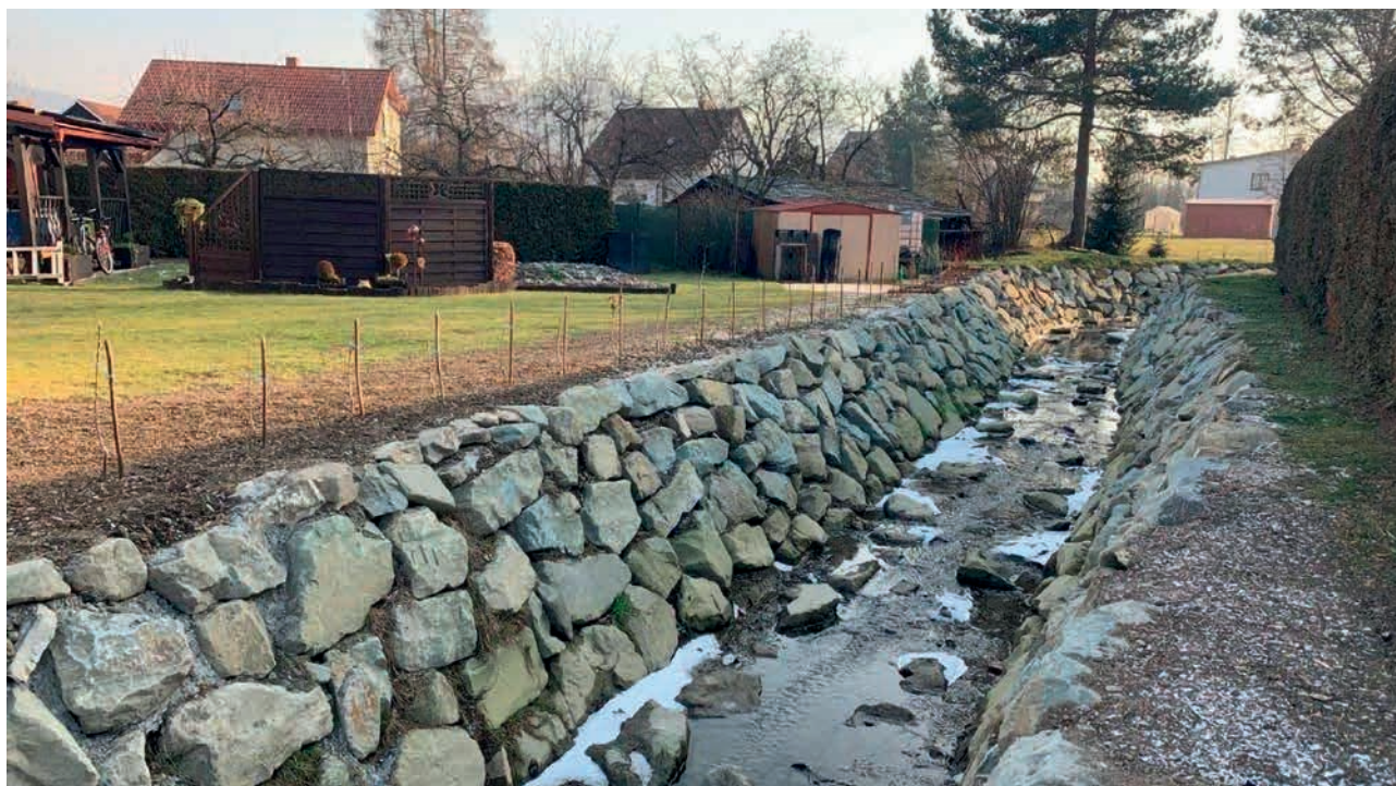
Anti-flood measures in the village of Fryčovice in the district Frýdek-Místek (source: Forest of the Czech Republic, s.e.)
