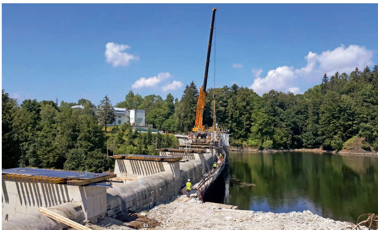
Reconstruction of the crown, The Pastviny Dam (source: Labe River Board, s.e.)
