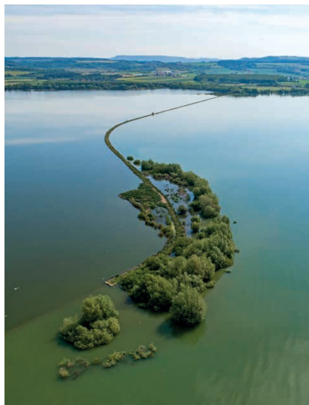
The Rozkoš Dam (source: Elbe River Basin, s.e.)
