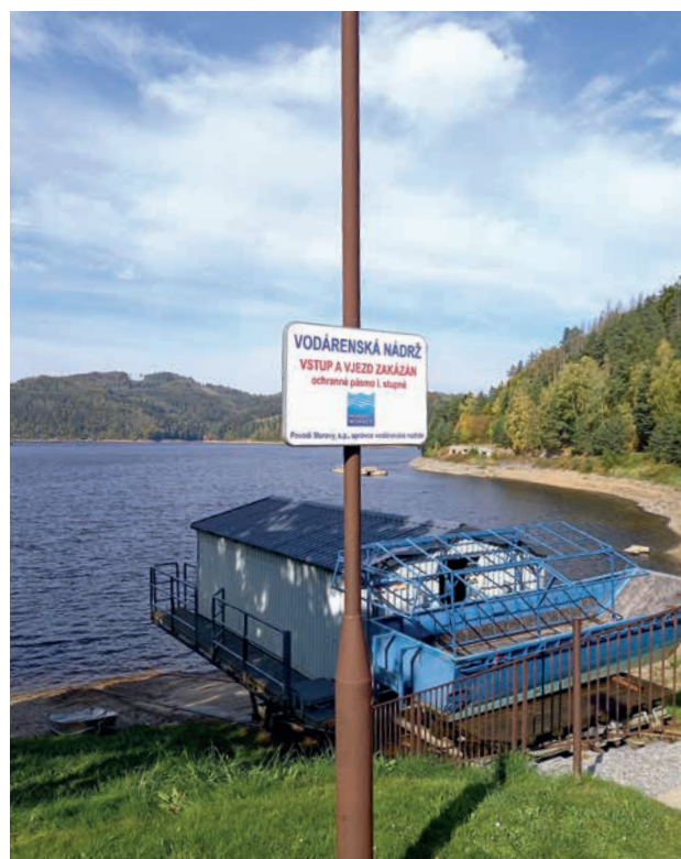
End of Work, the October 2021, the Vir Dam (author: Kopřivová Zuzana)
