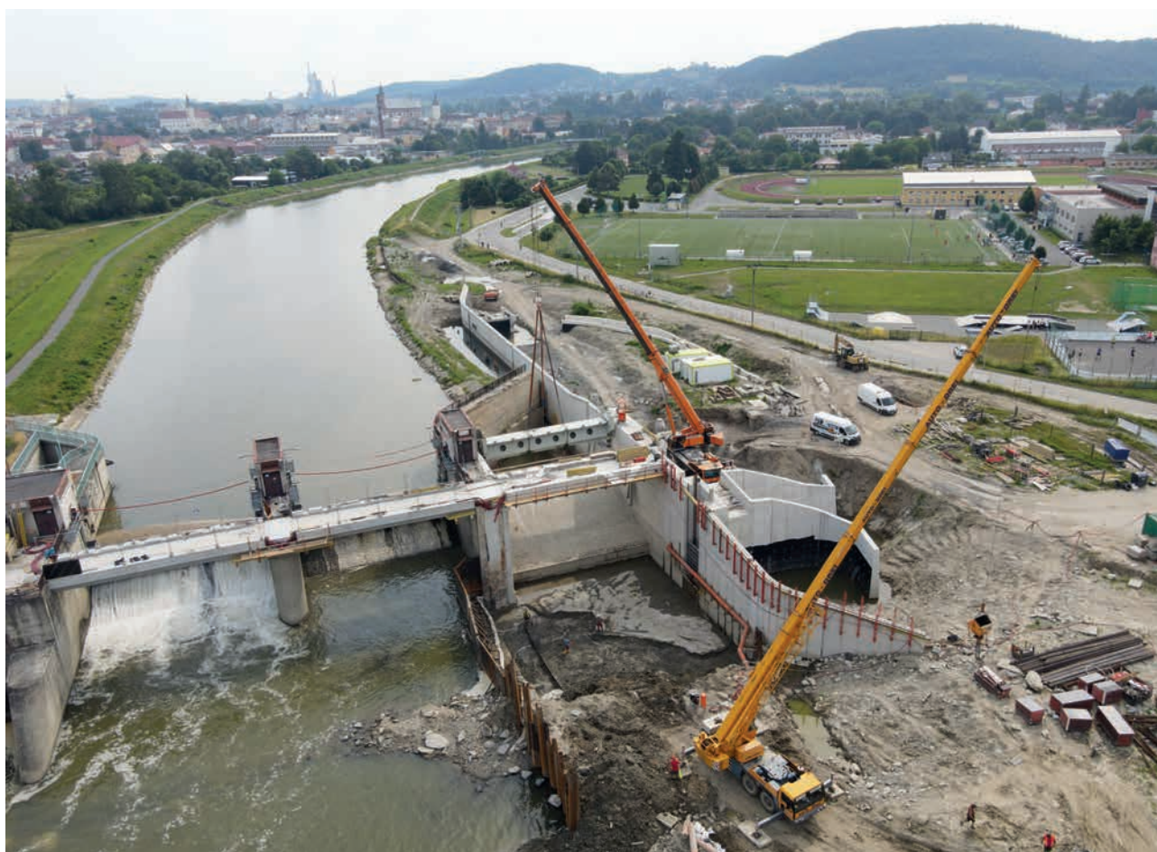
The Hranice Weir, progress of construction, June 2021 (source: Morava River Board, s.e.)
