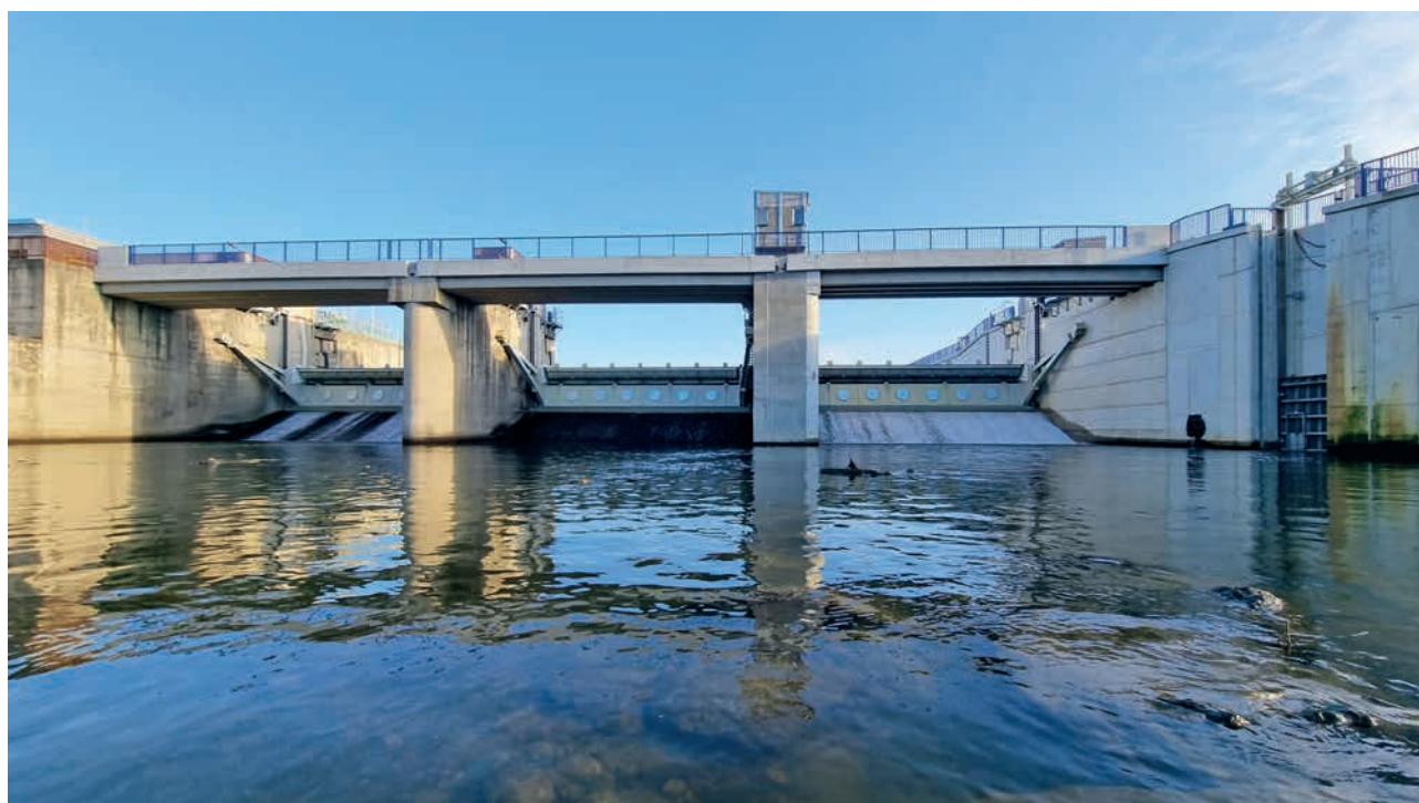
The Hranice Weir after completion, January 2022 (source: Morava River Board, s.e.)
