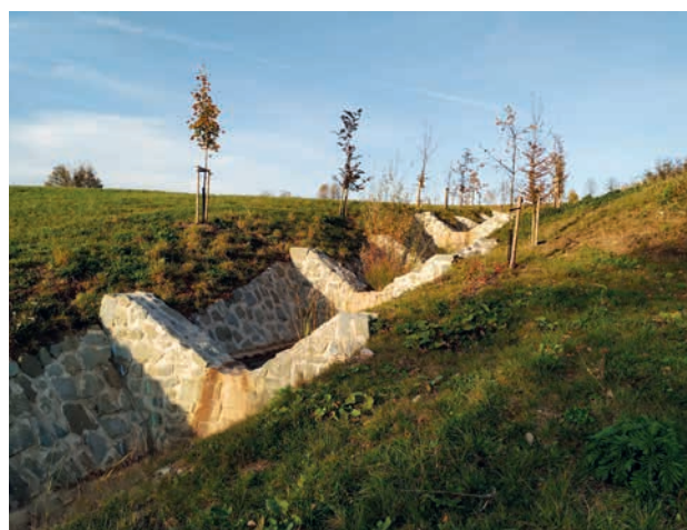
Drainage ditch with retarding elements and accompanying greenery in the cadastral area Třanovice (source: State Land Office)
